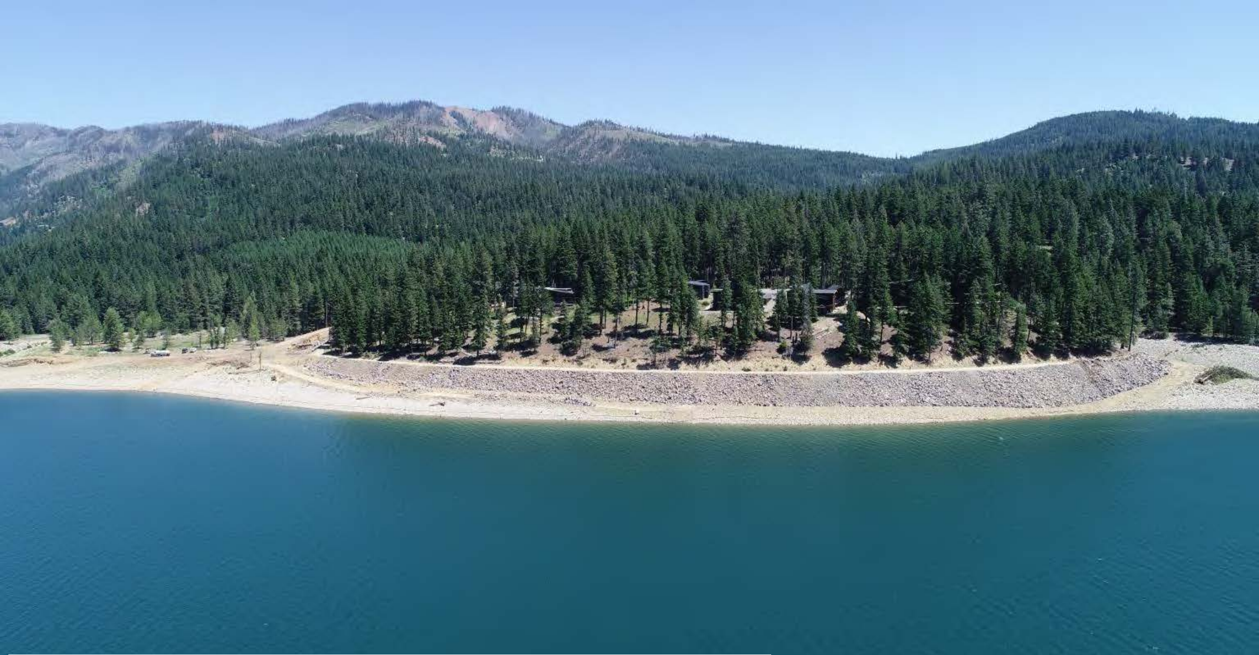
Timber Cove Shoreline Protection Facility – Under Construction
