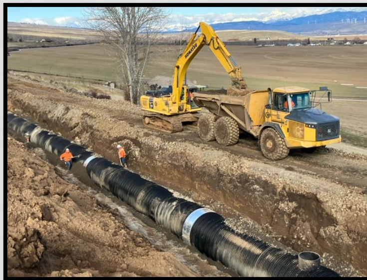
Kittitas Reclamation District South Branch Canal March 2024
