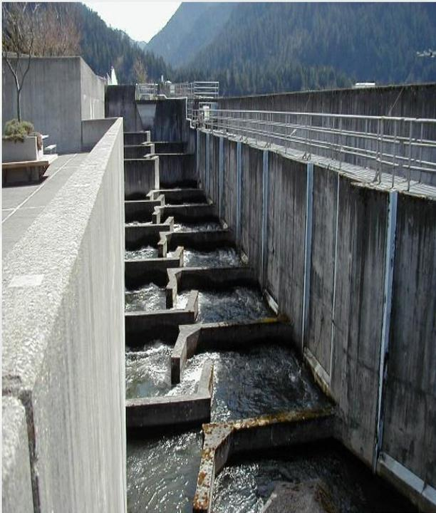
Vertical slot & orifice configuration
