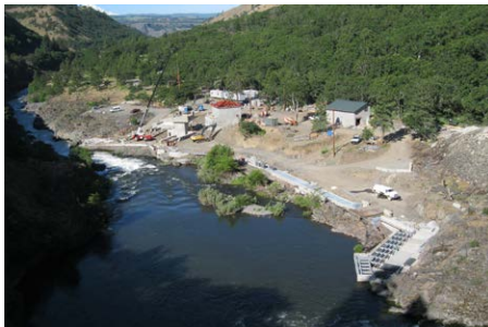
Lyle Falls Passage Facility, Klickitat River
