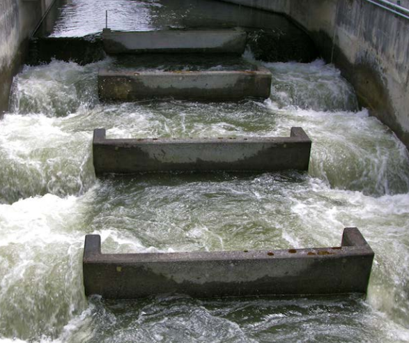
One of many types of fish ladders at Bonneville Dam.
