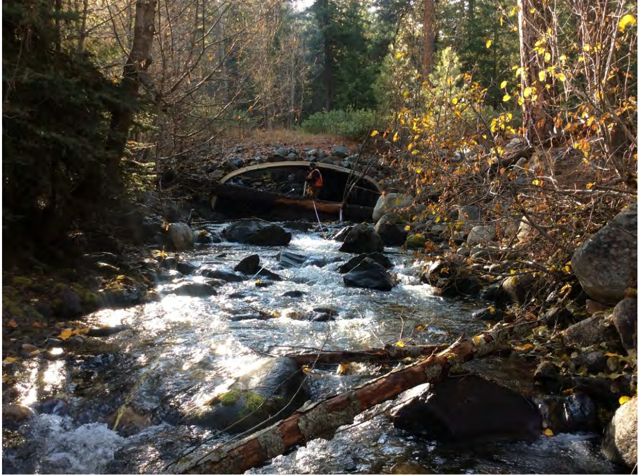
Figure 4-29. NF-4420 Road Crossing Culvert on Eagle Creek near RM 0.2
