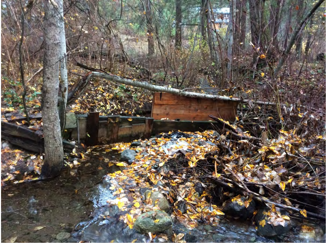
Figure 4-32. Water Diversion Structure on Canyon Creek near the Twisp River Confluence
