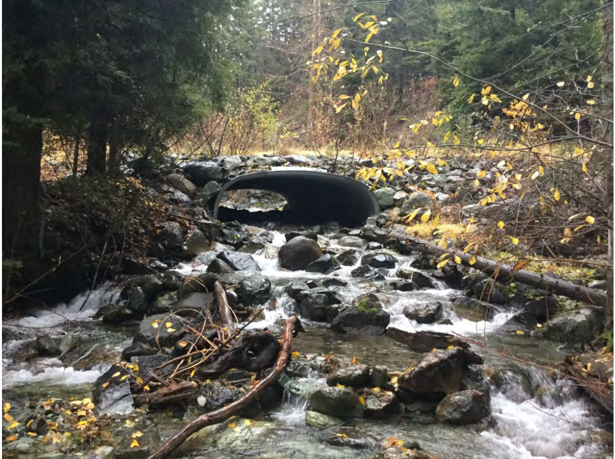
Figure 4-17. NF-4440 Road Crossing Culvert on North Creek near RM 0.5
