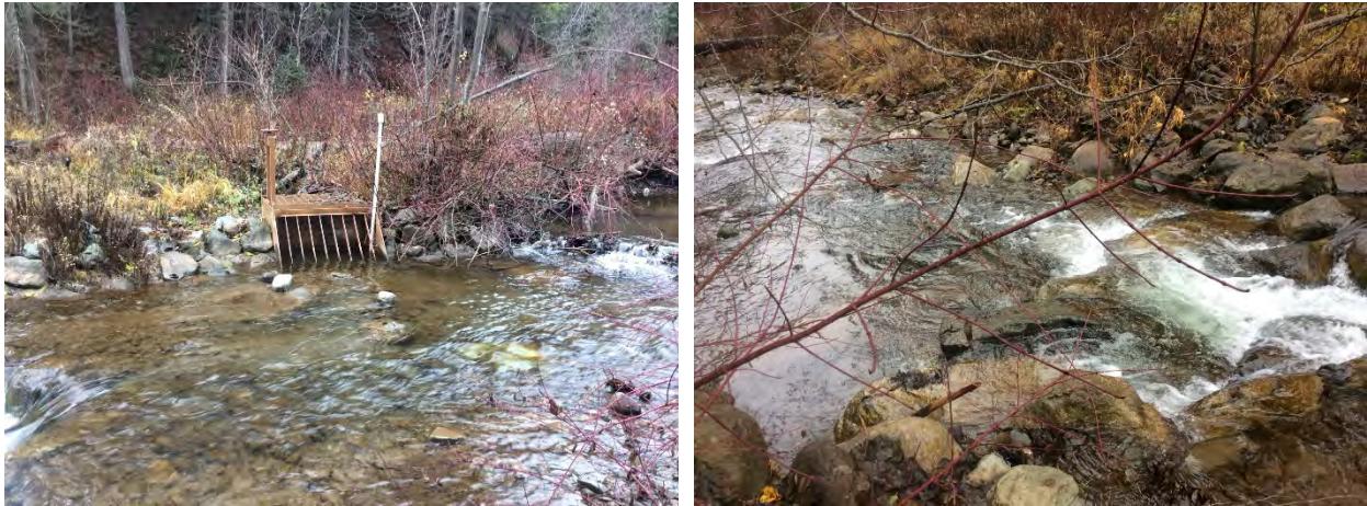
Figure 2-3. Photographs of Intake (left panel) and Rock Weir (right panel) Diversion in Little Bridge Creek Reach 2 near RM 2.2
