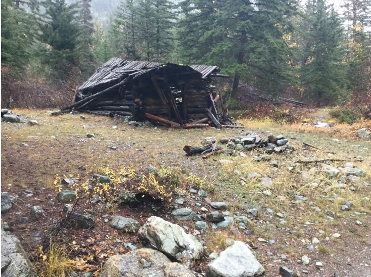
Figure 2-2. Photograph of Gilbert Mining Camp Cabin
