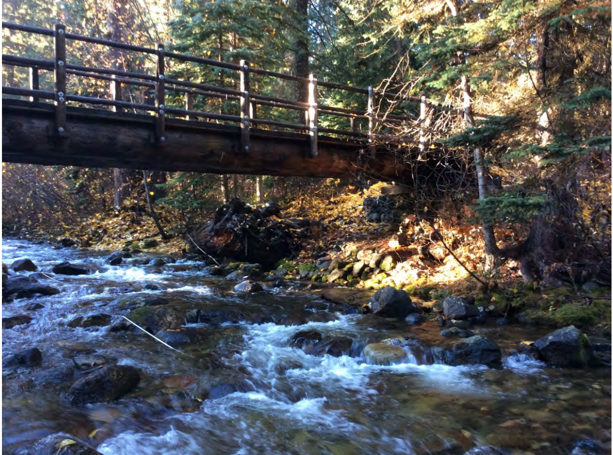
Figure 4-20. Pedestrian Bridge on the South Creek Trail near RM 0.3
