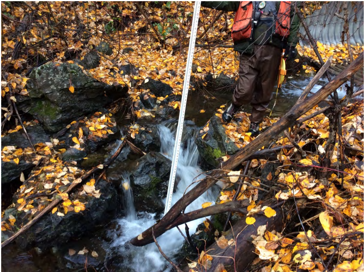
Figure 4-31. Riprap Drop Downstream of Twisp River Road Culvert near RM 0.2
