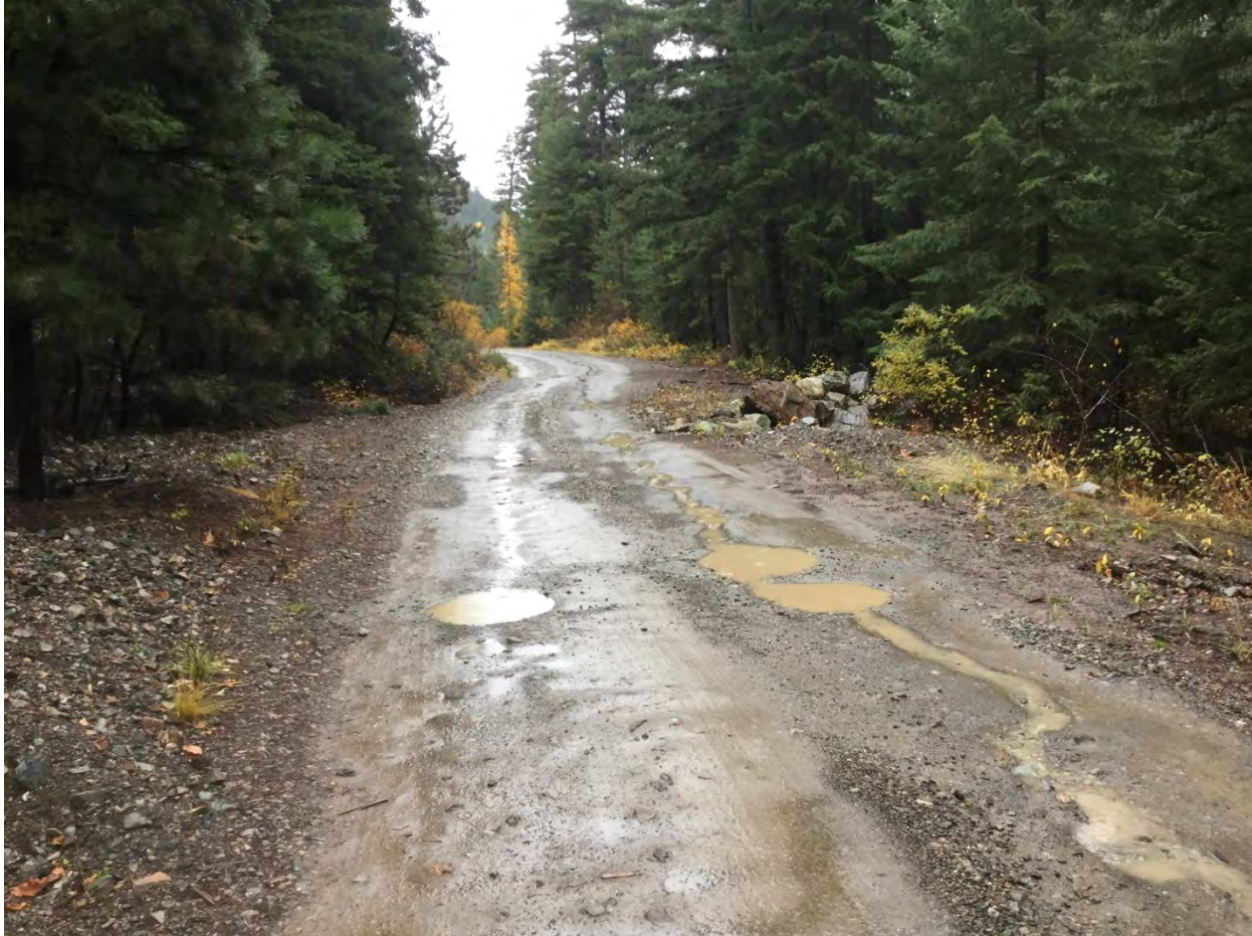
Figure 2-4. Photograph of Repaired Road Erosion on the NF-4440 Road near RM 23.7
