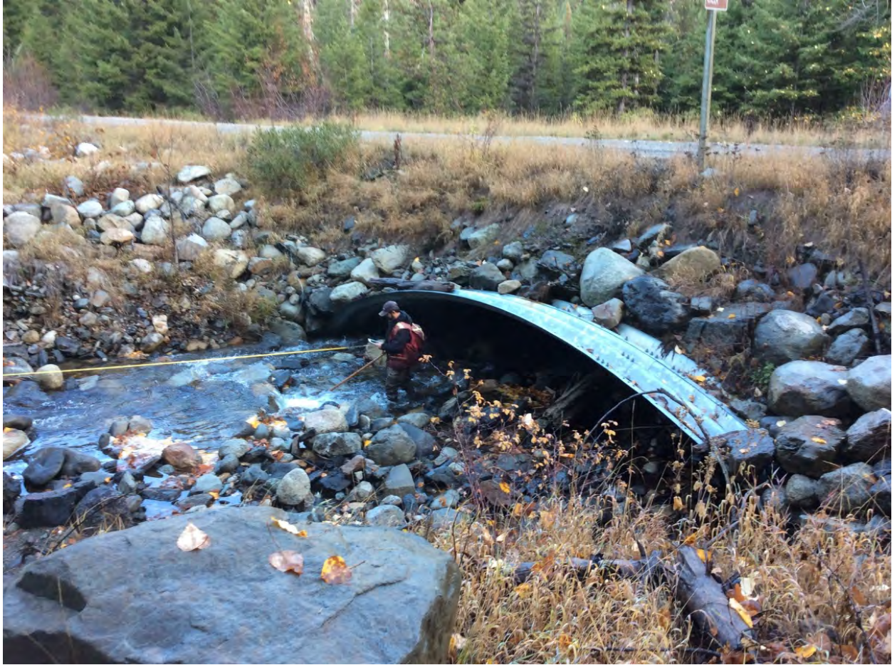
Figure 4-23. NF-4435 Road Crossing Culvert on Reynolds Creek near RM 0.1
