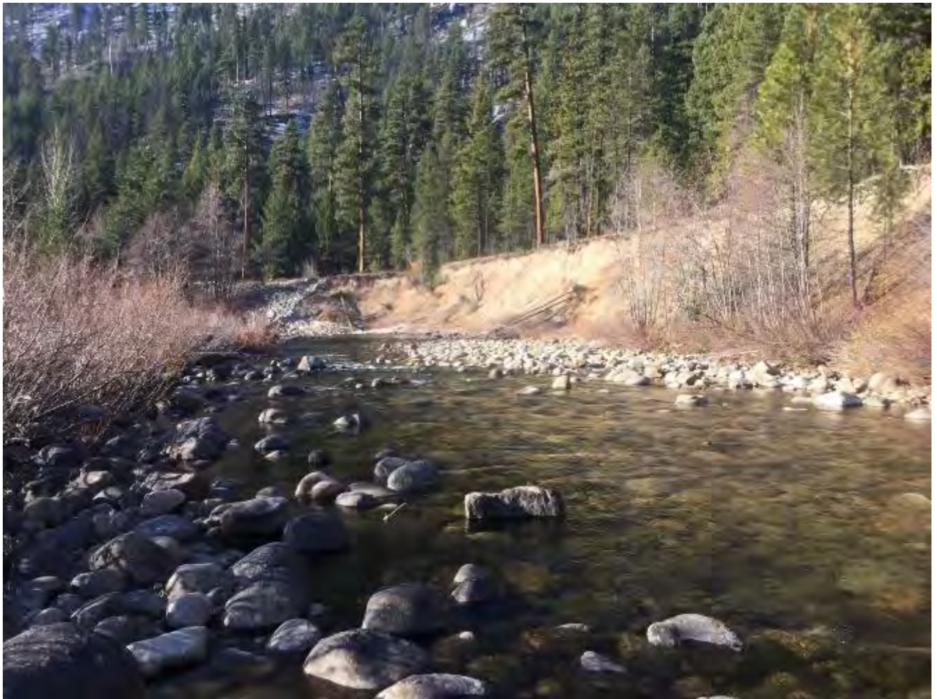
Figure 27. Significant active bank erosion at RM 21.8 threatens USFS Road 5160.
