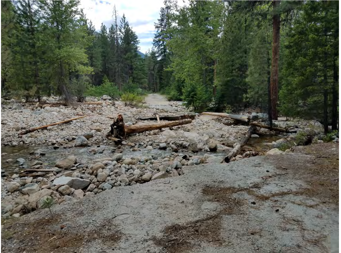
Figure 49. Partially washed out fish barrier on Twentymile Creek at the USFS Road 5010 ford (RM 0.1).
