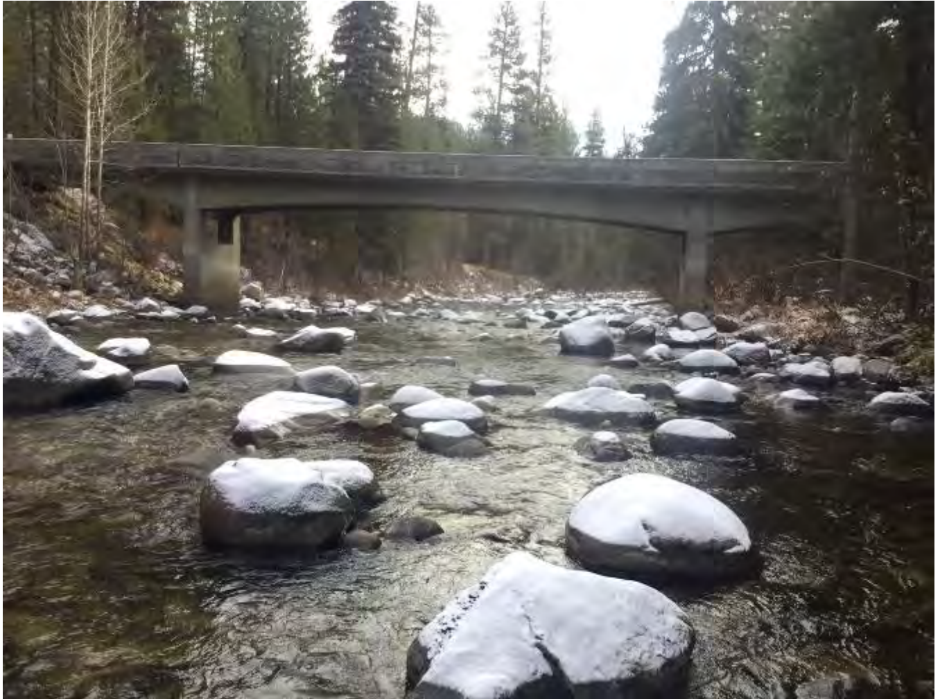
Figure 9. Bridge over the Chewuch River at RM 20.4.
