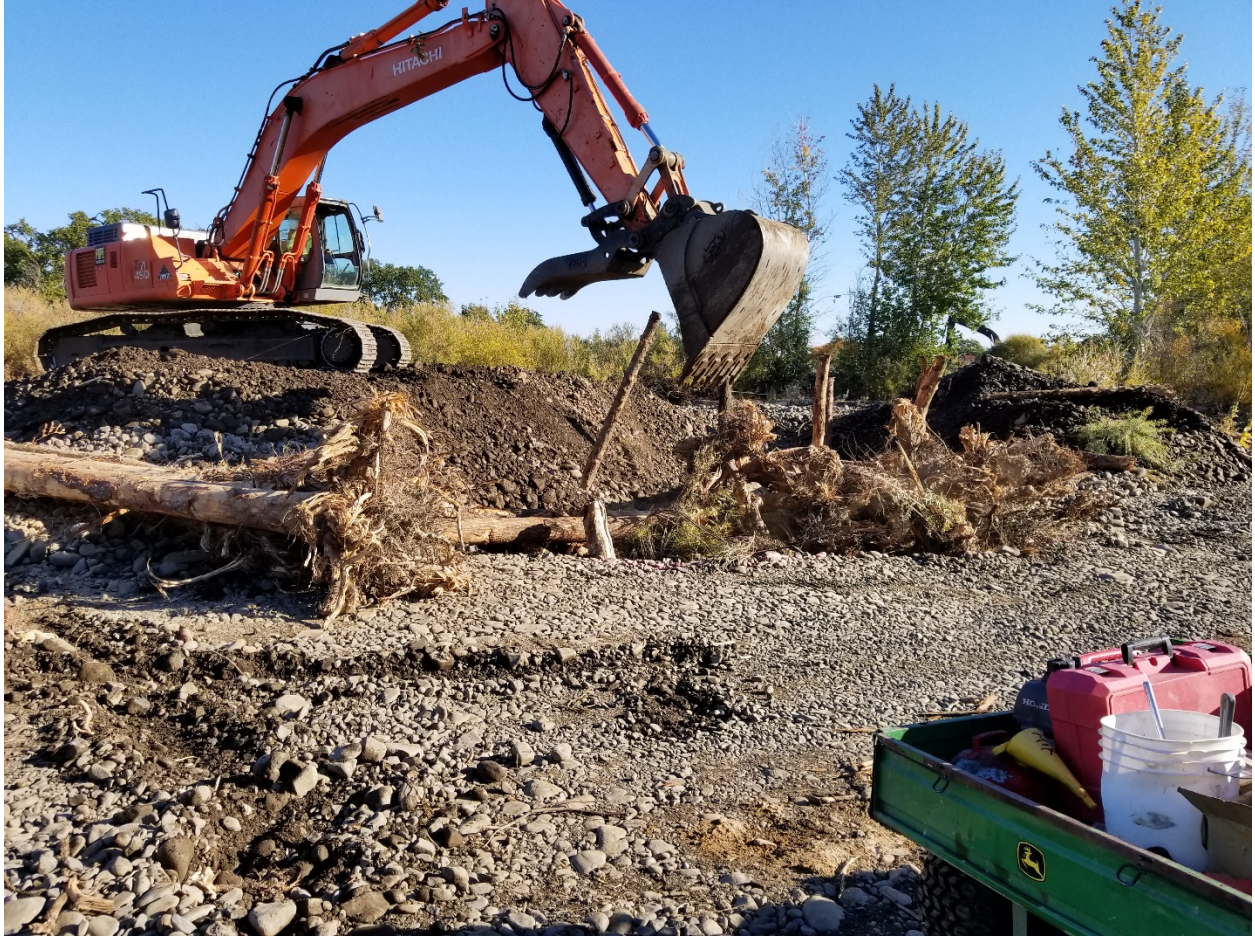
Figure 4. Construction of a large engineered log jam (ELJ) for bank stabilization at the lower end of the 3-Way Levee removal project site.
