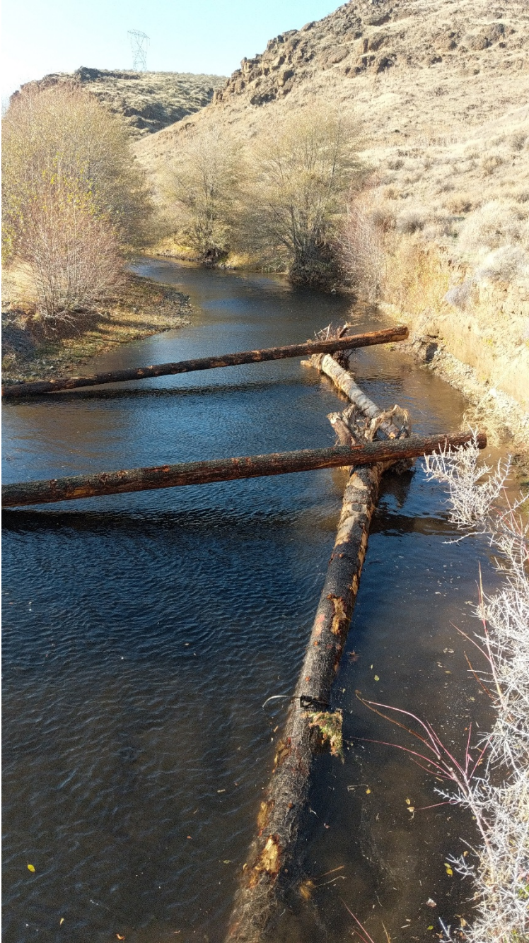
Figure 8. 2x structure designed to limit pressure on the exposed and eroded right bank.
