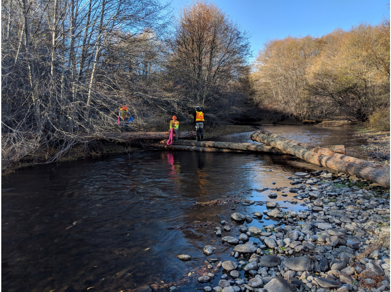
Figure 7. Channel spanning structure designed to forces water out of stream channel and onto floodplain and riparian zone.
