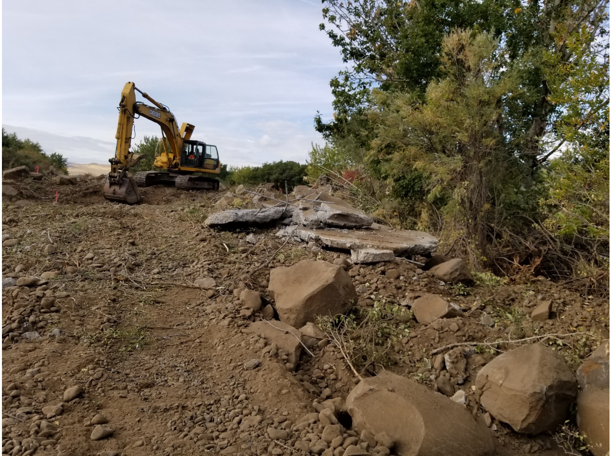
Figure 1. Removal of the 3-way irrigation diversion structure.
