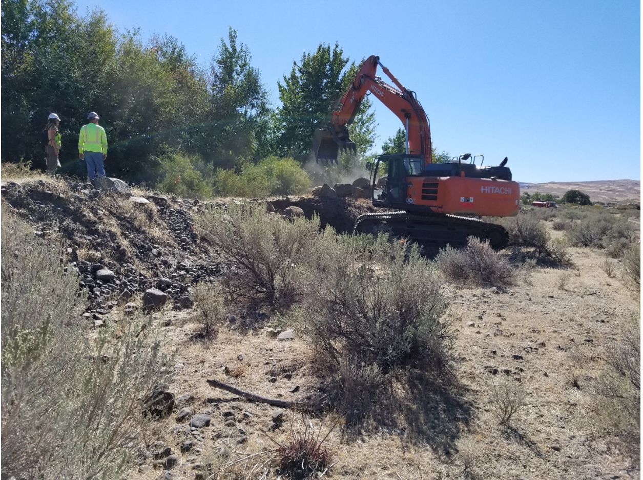
Figure 2. Removal of the 0.3 mile section of levee upstream from the diversion structure.
