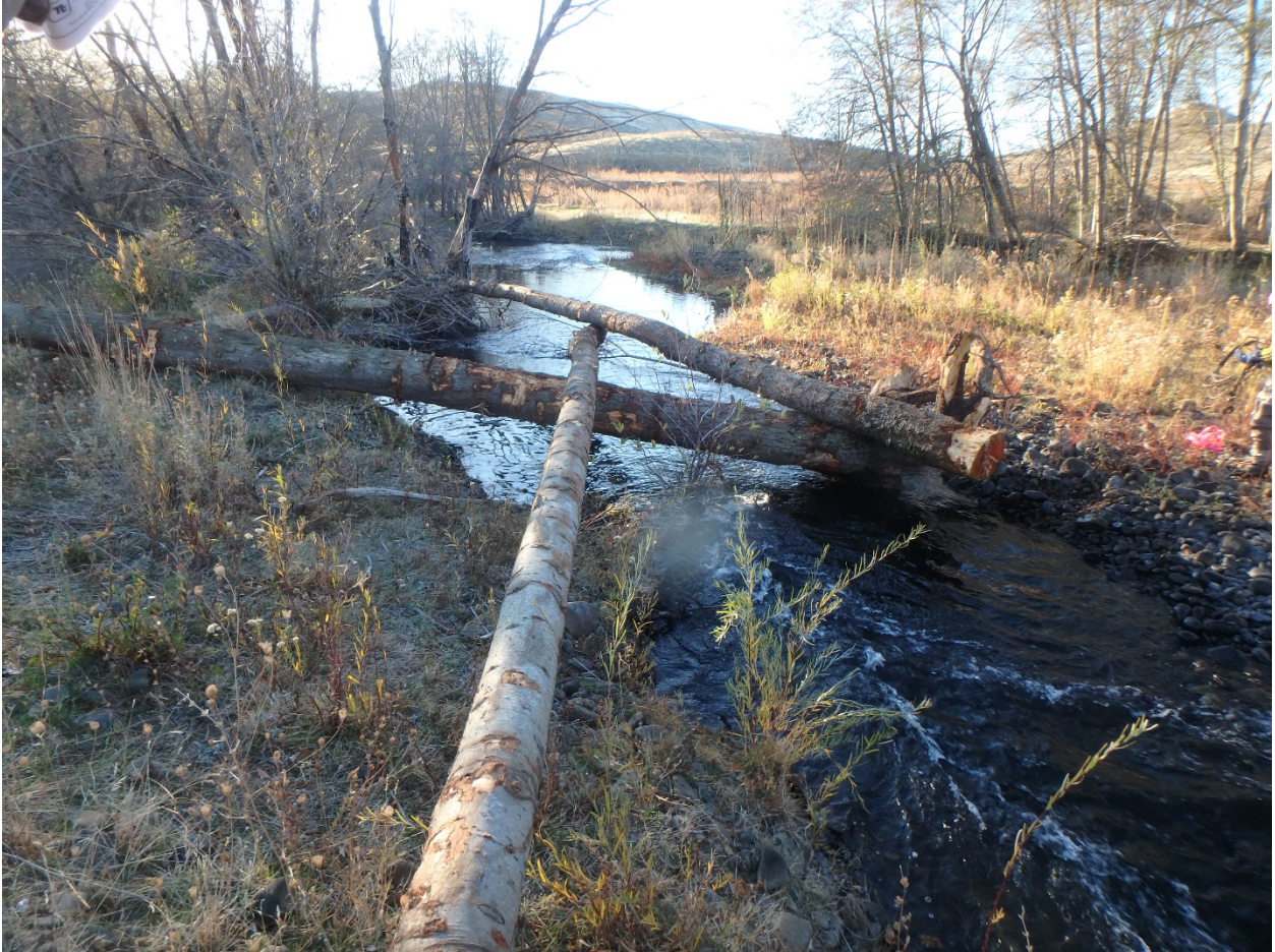
Figure 9. Example of 3x Structure. Includes one (1) root wad and two (2) logs. Designed to relieve banks of high stream energy.
