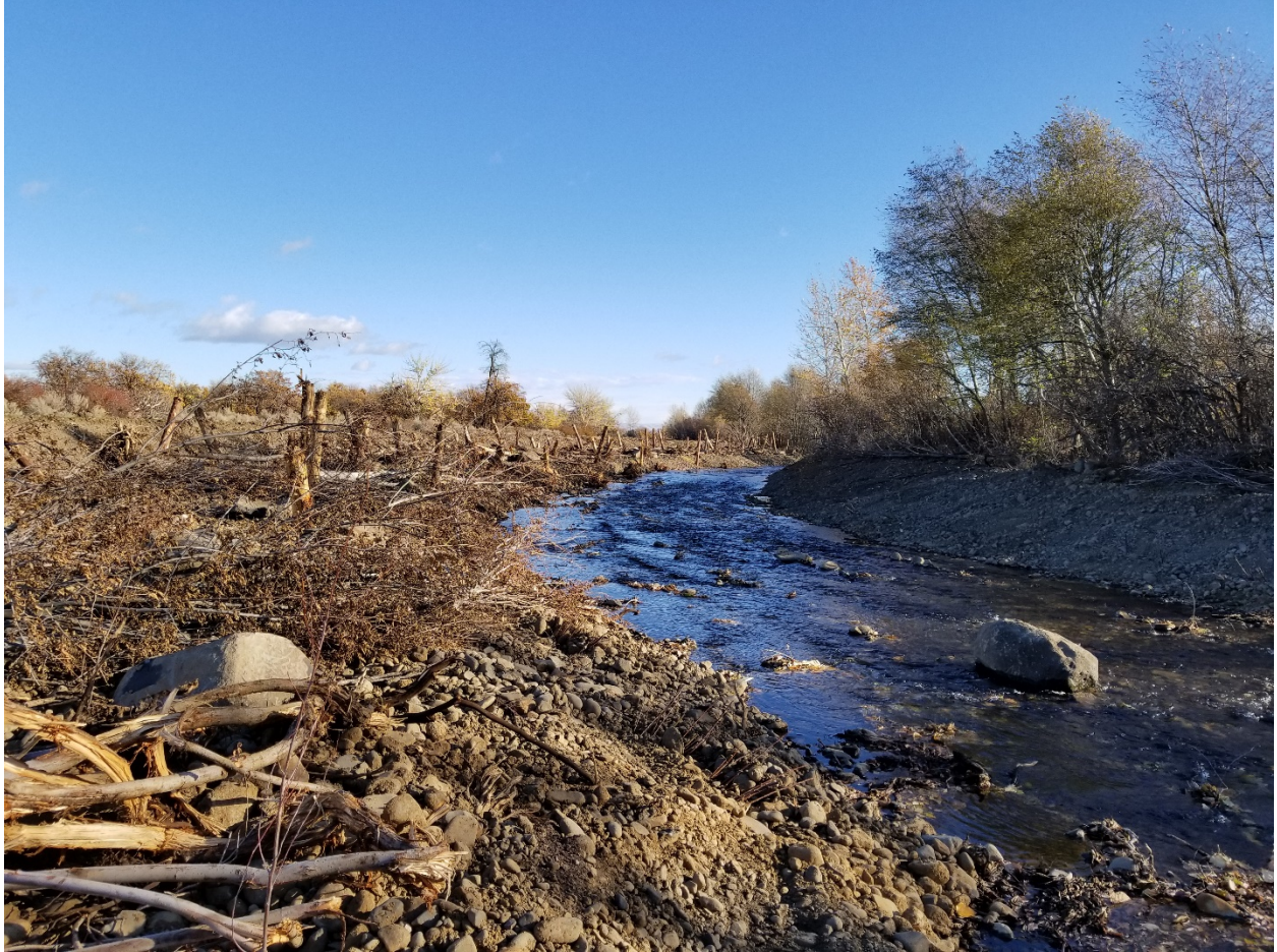
Figure 3. Newly constructed stream channel of Toppenish Creek and inset floodplain in the location where the 3-Way Levee was removed.
