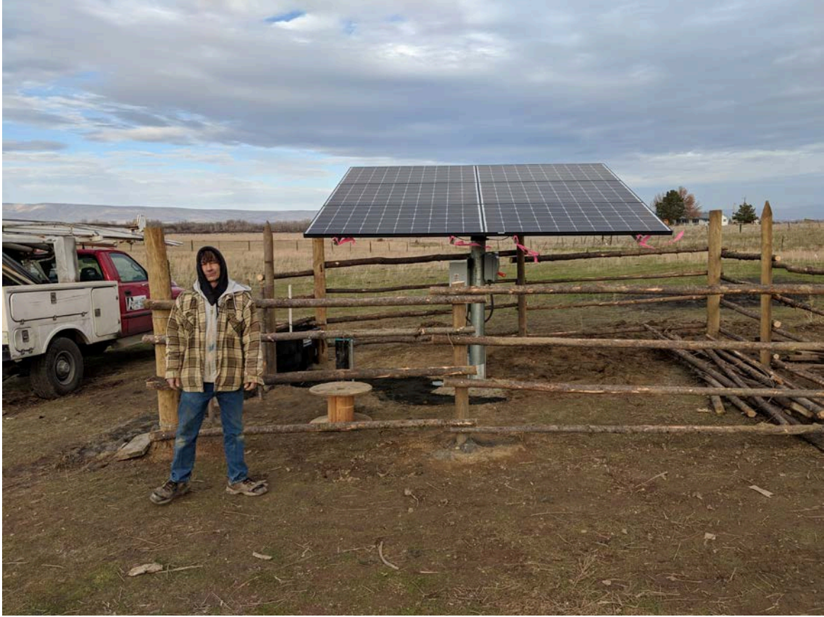
Figure 5. Solar Panels, fence and stock water tank, completed.
