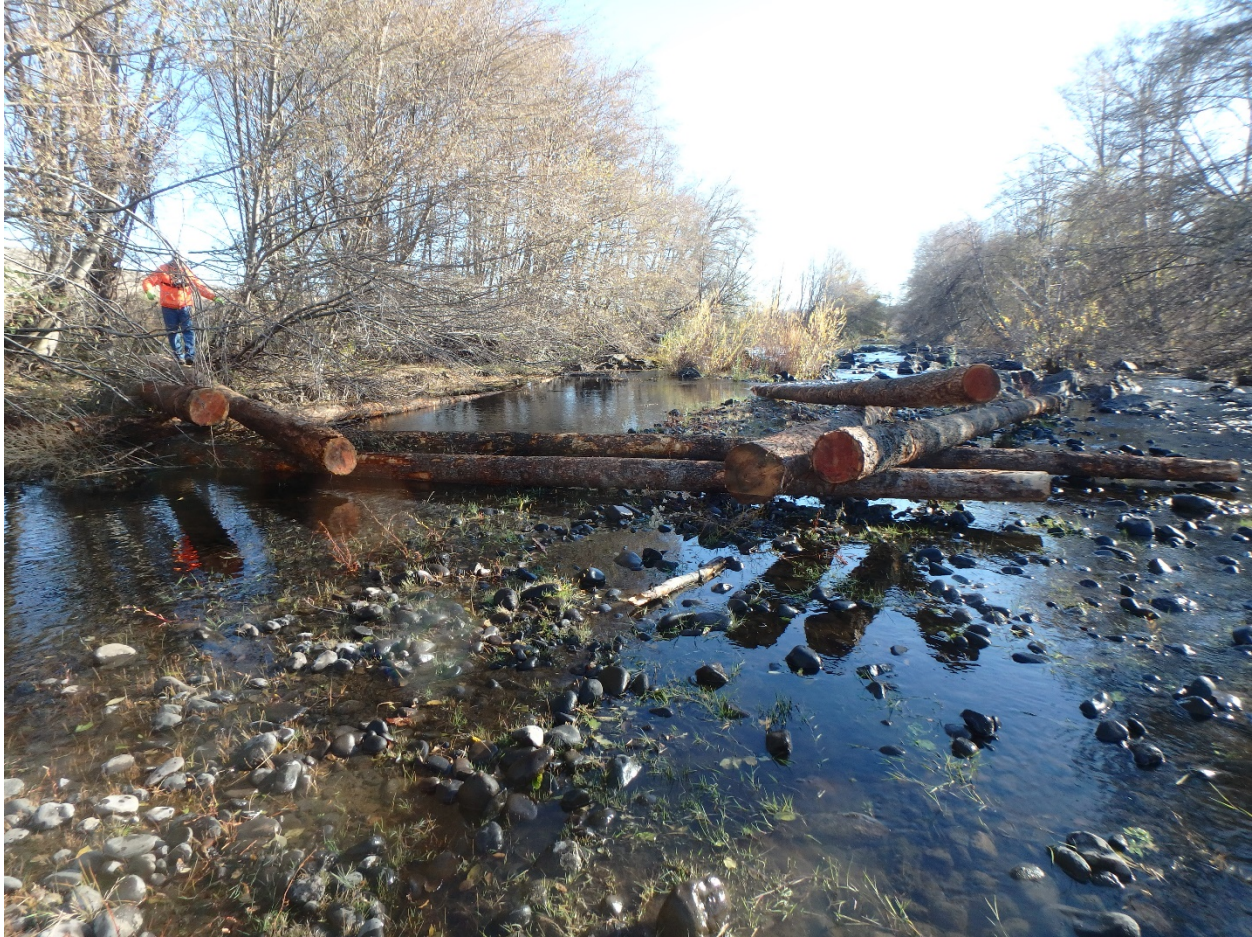
Figure 10. 7 log structure for retaining water in a back-water setting after a high low event.
