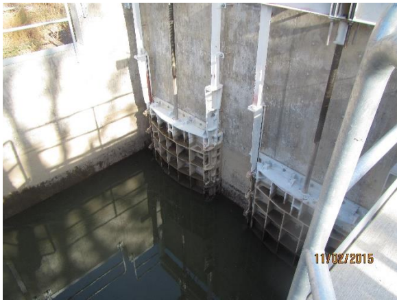
Photo 2. The regulating gates after dewatering looking downstream (left photo). The regulating gates after dewatering looking upstream (right photo). In 2018, the gates were fully shut after the reopening of the headgates for the winter months. Water level is generally low after irrigation shutdown, limiting potential damages caused by freezing water coming into contact with the gates.
