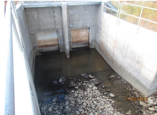
Photo 2. The regulating gates after dewatering looking downstream (left photo). The regulating gates after dewatering looking upstream (right photo). In 2018, the gates were fully shut after the reopening of the headgates for the winter months. Water level is generally low after irrigation shutdown, limiting potential damages caused by freezing water coming into contact with the gates.
