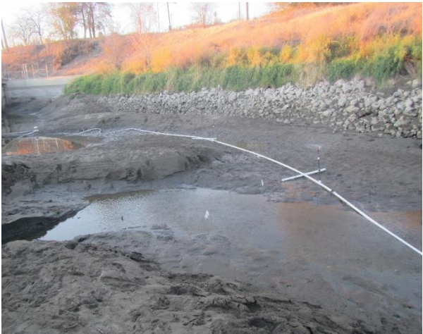
Photo 2. Overview of the sprinkler system operation downstream of the fish screens at Sunnyside Diversion immediately after dewatering occurred. Part of the sprinkler system covers the high density isolated pools.
