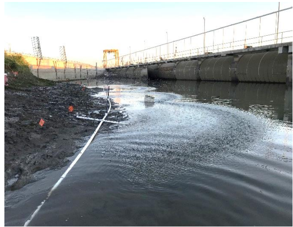
Photo 1. Overview of the sprinkler system operation upstream of the fish screens at Wapato Diversion immediately after dewatering occurred (left photo). In the right photo, the sprinkler spray is submerged to some extent in the large water body because we were not certain how far the water level was going to drop overnight (and what new sediment would become exposed).
