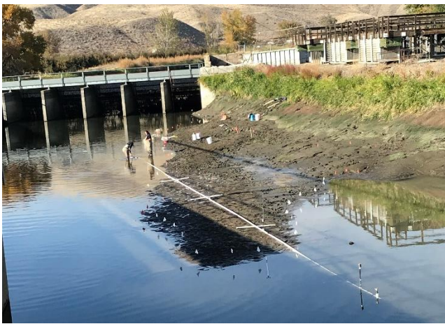
Photo 1. Overview of the sprinkler system operation upstream of the fish screens at Wapato Diversion immediately after dewatering occurred (left photo). In the right photo, the sprinkler spray is submerged to some extent in the large water body because we were not certain how far the water level was going to drop overnight (and what new sediment would become exposed).
