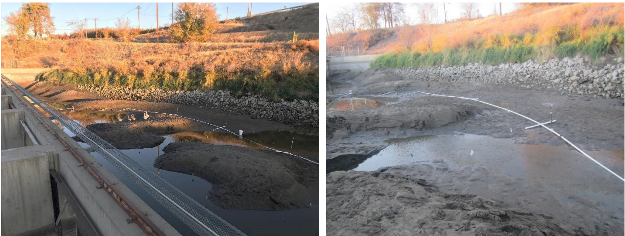
Figure D3-2. Overview of the sprinkler system operation downstream of the fish screens at Sunnyside Diversion immediately after dewatering occurred. Part of the sprinkler system covers the high density isolated pools.
