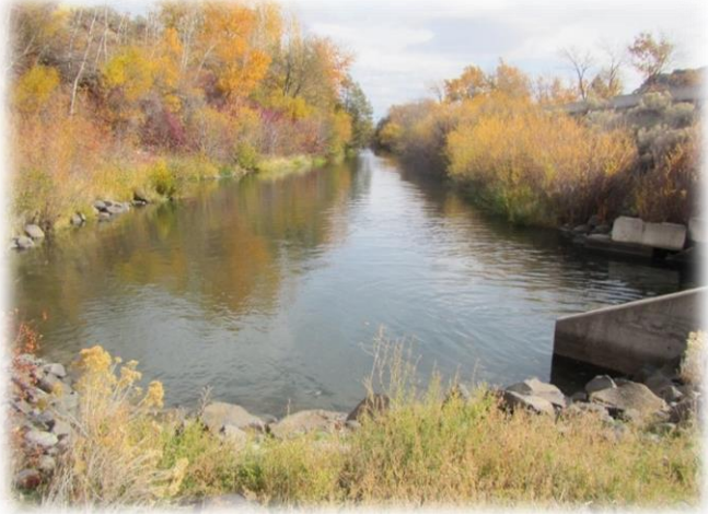
Photo D4. Downstream view of the Wapatox Diversion irrigation canal (Naches River), immediately downstream of the headgates.
