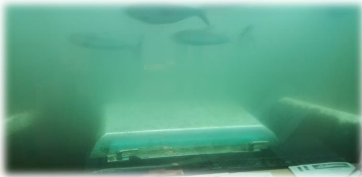
Photo K1. Lamprey resting boxes installed in front of the public viewing window at Bonneville Dam Washington Shore Ladder with one adult lamprey attaching to the window on June 27, 2018.
