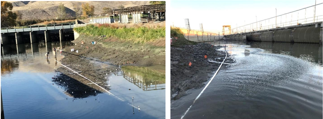
Figure D3-1. Overview of the sprinkler system operation upstream of the fish screens at Wapato Diversion immediately after dewatering occurred (left photo). In the right photo, the sprinkler spray is submerged to some extent in the large water body because we were not certain how far the water level was going to drop overnight (and what new sediment would become exposed).
