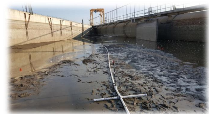
Photo D3. Sprinkler system set up at Wapato Diversion upstream of the fish screens to help maintain the dewatered fine sediment wet overnight on October 19, 2018.
