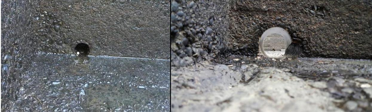
**Figure 7. Photos of the drainage holes at Roza Dam. Left photo is the original 2 inch hole, and the right photo is the new 4 inch holes.**
