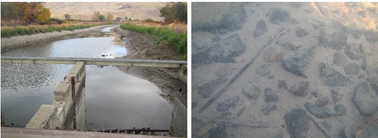
Photo 2. Overview photo of the upstream canal at Wapato Diversion (left photo) and a close-up of the habitat (silt and cobble substrates) where freshwater mussels have been found (right photo).
