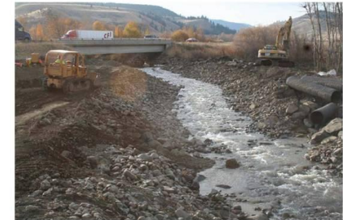
AFTER: Removal restores fish passage
