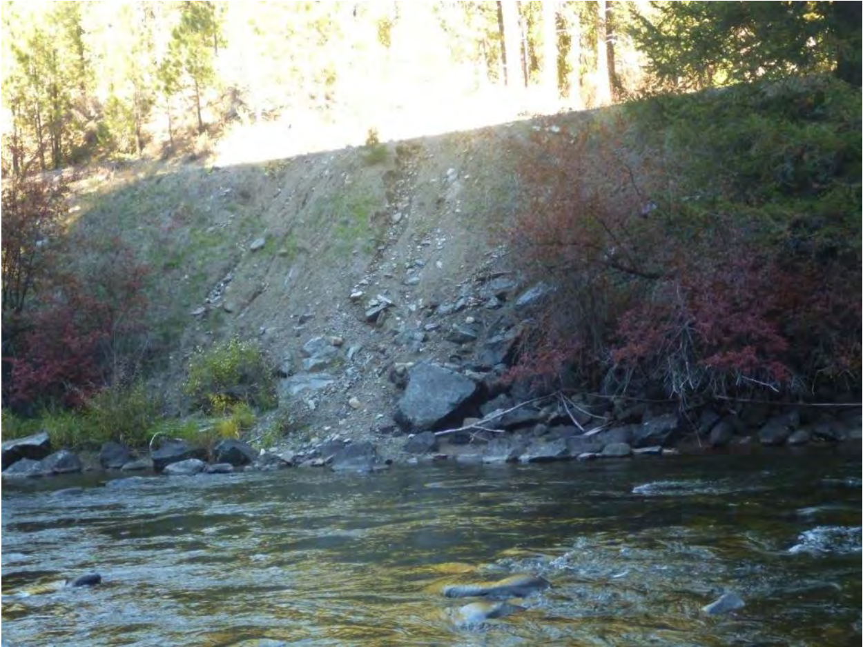
Figure 32 The roadway on river-left acts as a source for fine sediment, sand, and gravel entering the channel.
