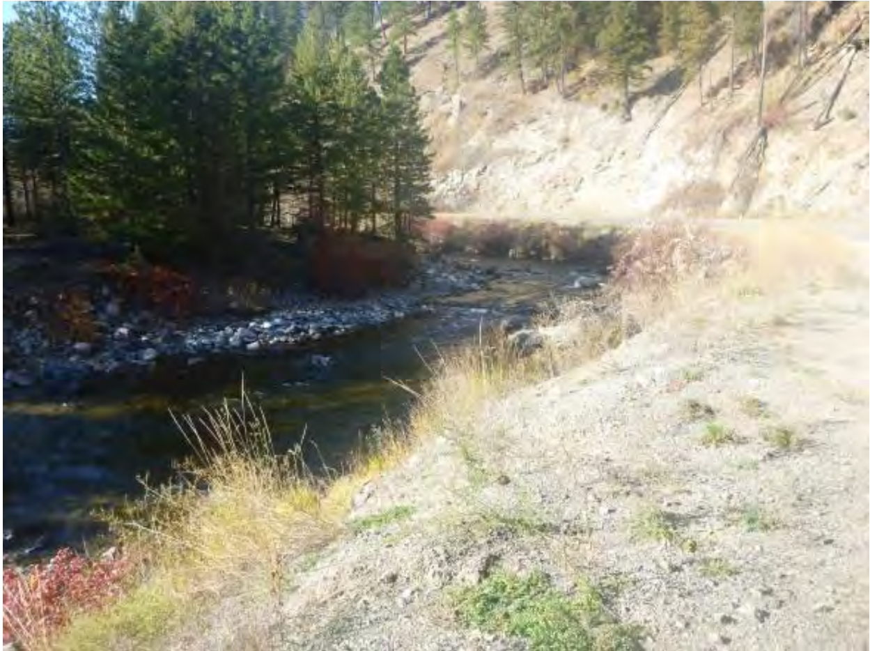
Figure 36 The road embankment at RM 9.15 looking upstream.
