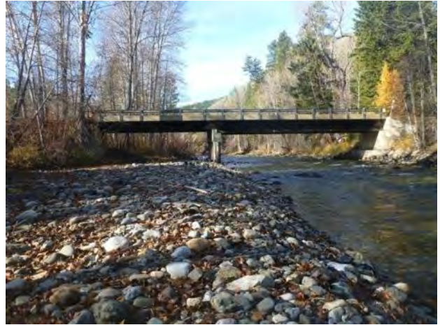
Figure 61. Bridge at RM 13.5 looking upstream.
