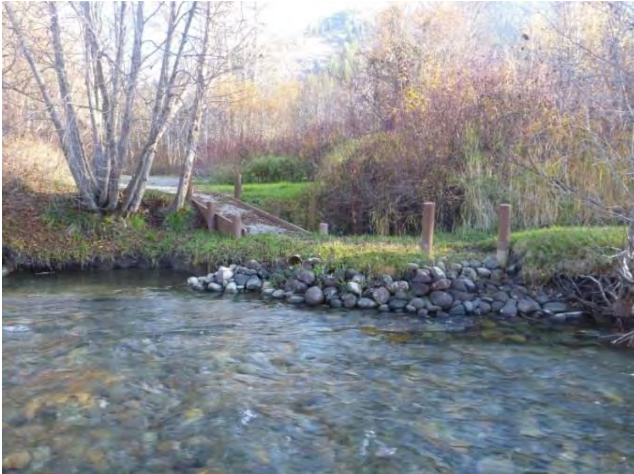
Figure 76. RM 13.8 riprap with large posts and a constructed footbridge constructed along river right opening to a gravel clearing.
