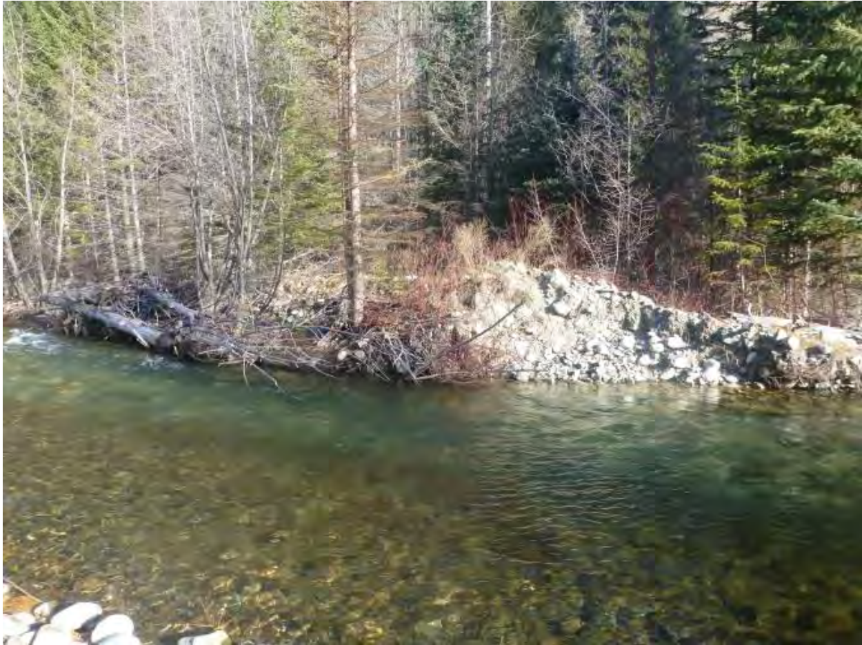
Figure 93. The push-up levee on river left at RM 16.8 is composed of cobbles and sands.
