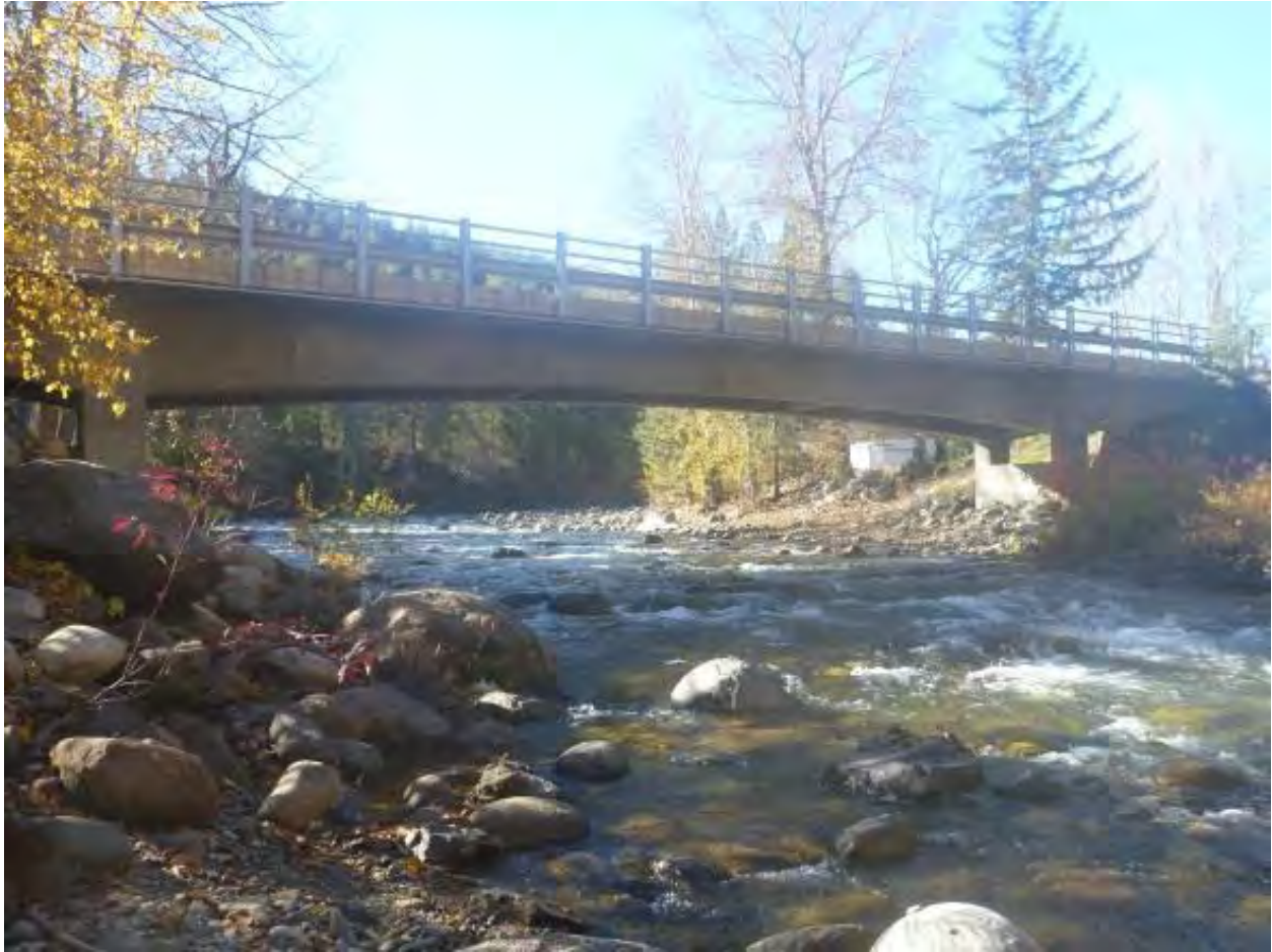
Figure 23 Looking upstream at the bridge at RM 8.4.
