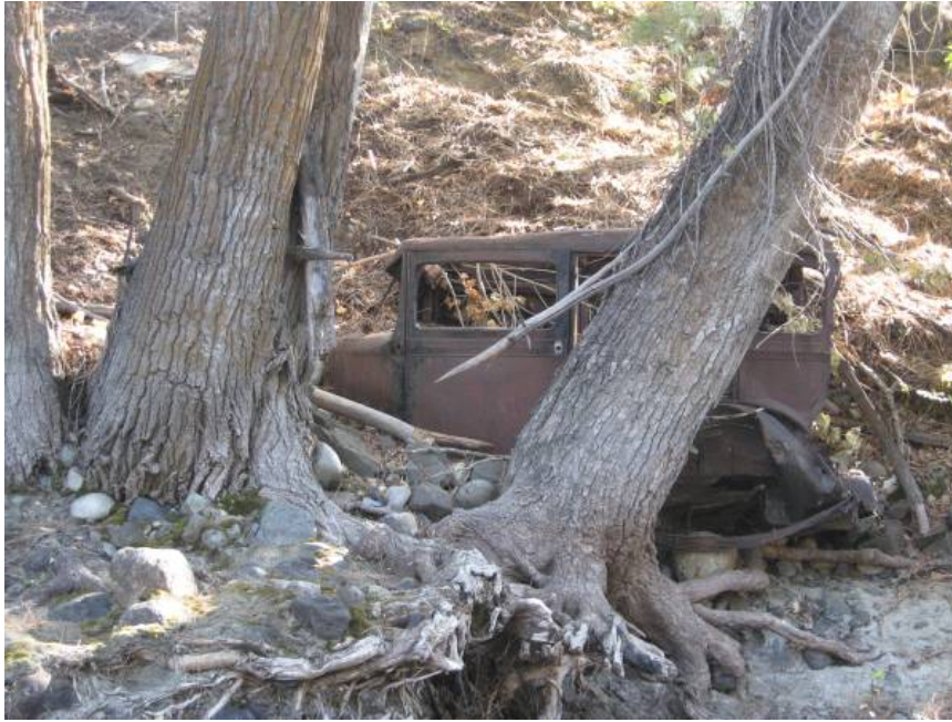
Figure 13. Old car bodies (“detroit riprap”) have been incorporated into streambanks in several locations (October 2009).
