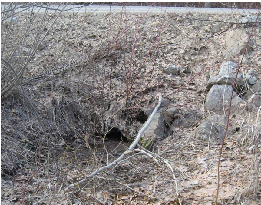
Figure 41. Culvert (mostly plugged) draining floodplain ponds at RM 1.95 (river-right bank) (March 2010).
