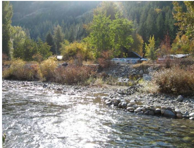
Figure 16. View looking downstream toward the west at the levee and development in the floodplain along river-right near RM 1.65 (October 2009).
