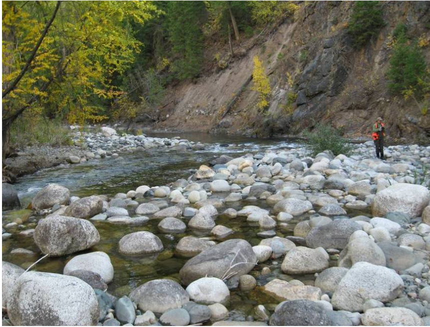
Figure 67. Exposure of bedrock and erosion of glacial material near RM 6.55 (October 2009).
