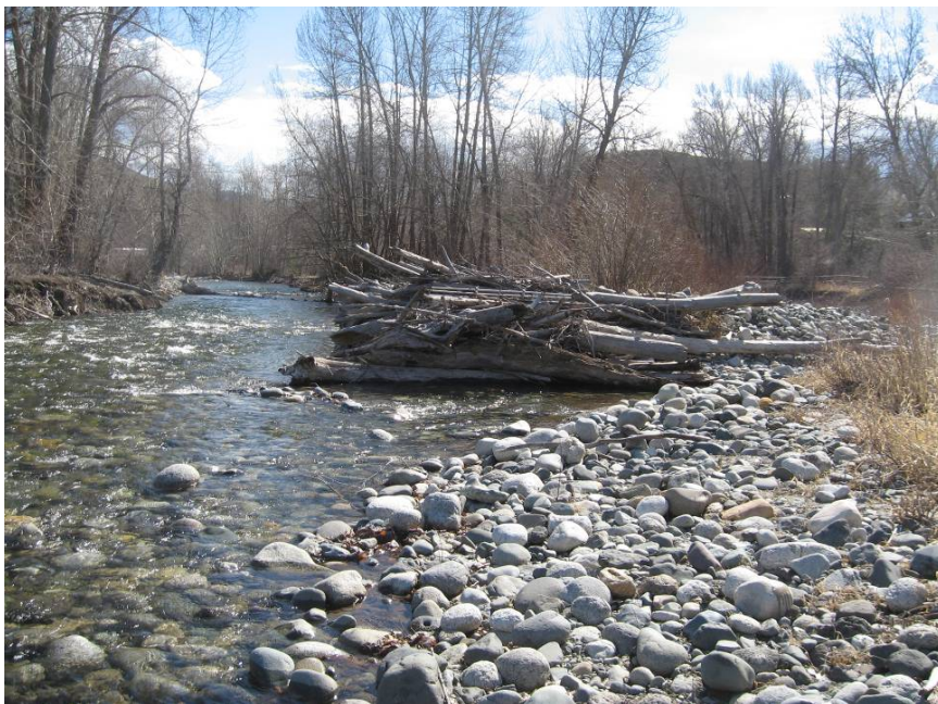
Figure 28. Constructed/enhanced bar apex log jam at RM 1.1 (March 2010).
