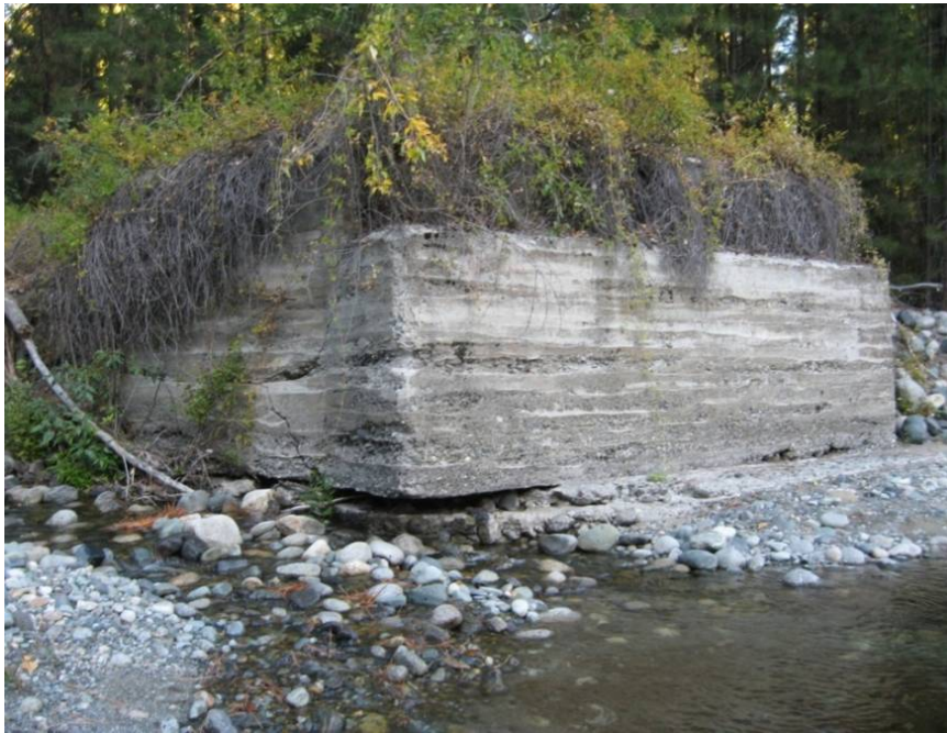
Figure 40. Old concrete footing/abutment near RM 1.9 (October 2009).
