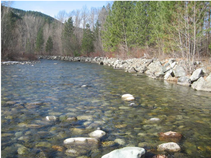
Figure 26. View looking upstream near RM 1.75 at riprap on river-left bank (March 2010).
