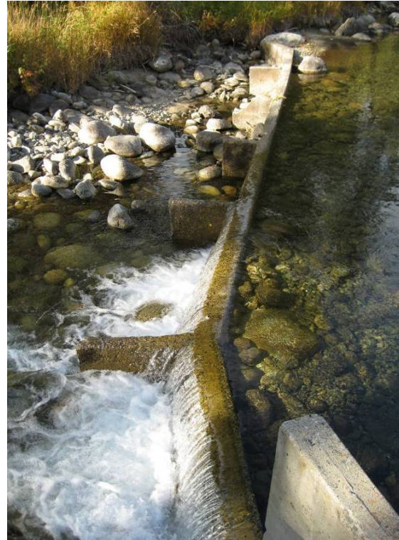
Figure 69. Concrete diversion weir at RM 7.6 used to divert flow into an irrigation canal (October 2009).
