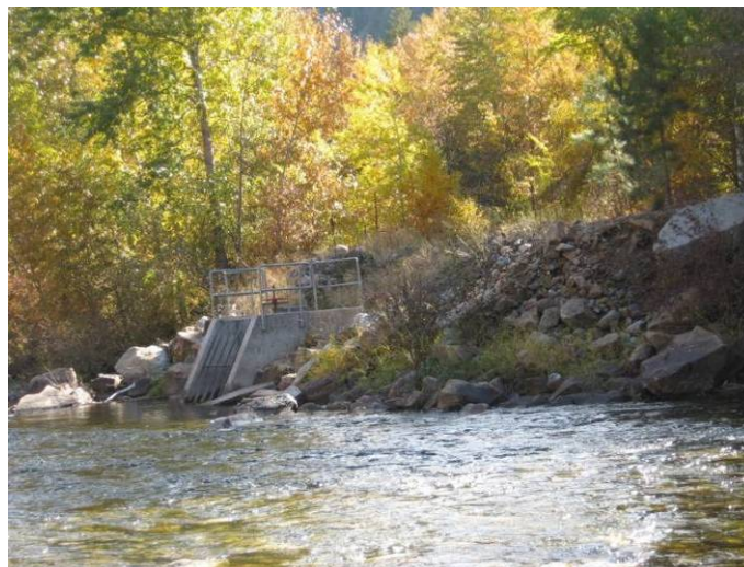
Figure 17. Diversion structure supplying surface water to restored off-channel ponds along the river-right floodplain (October 2009).
