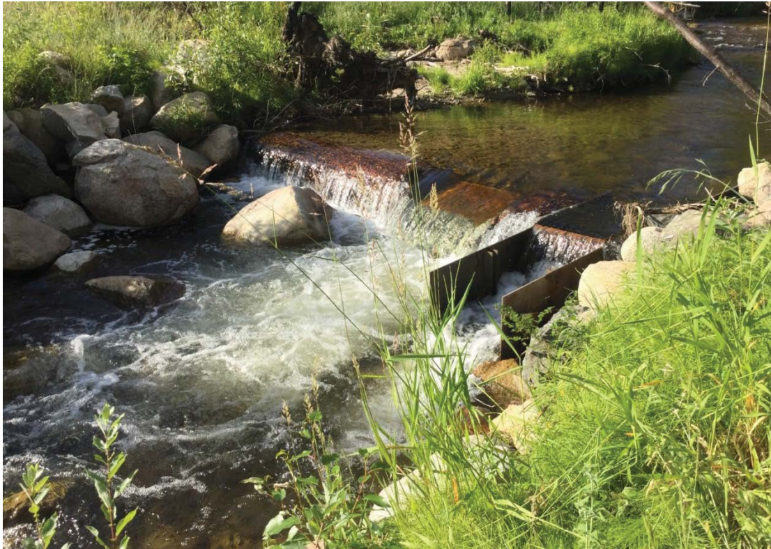
Figure 2-3. Photograph of Log Weir and Ladder Structure near RM 6.3 at Batie Diversion
