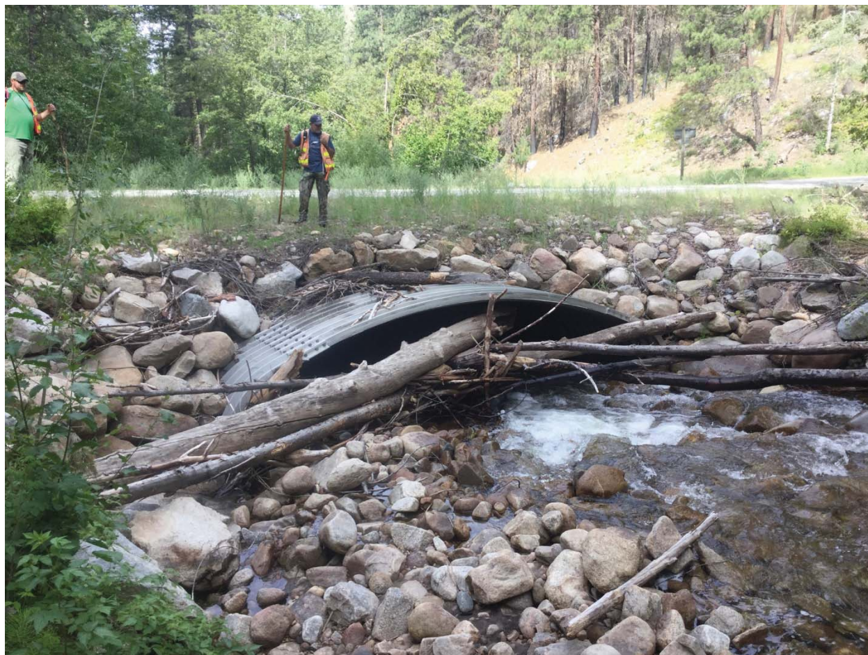
Figure 2-6. Photograph of Wood Racking at Culvert Crossing Inlet on NF-4225 Road near RM 9.5
