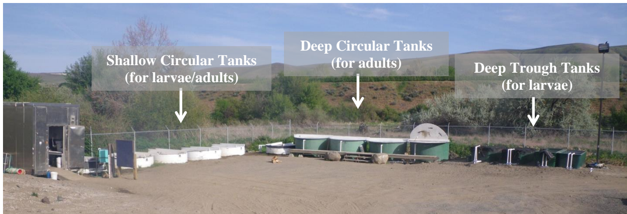
Figure 5-5. East Lamprey Facility at Prosser Fish Hatchery.
