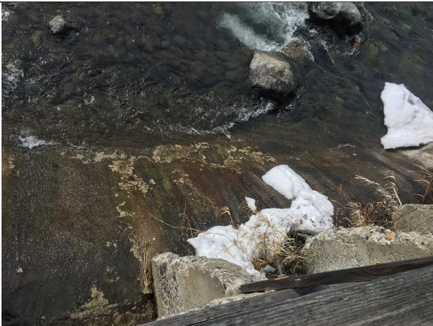
Section 1, upper bypass gate outlet on the Wenatchee River. (March 2, 2017)
