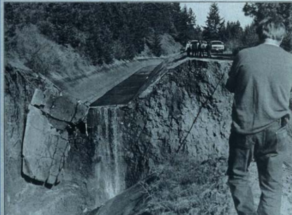
Officials surveyed the scene of the wrecked KRD Highline Canal this morning. The ruptured canal released a wall of water that wiped out power and telephone lines. Irrigation water deliveries will be delayed until the canal is repaired, officials report.
