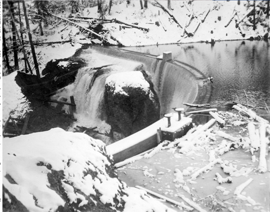
P33-A10YB-002 View of Clear Creek Dam shortly after completion, showing water flowing over crest. Photographer Unknown, c. 1912.
