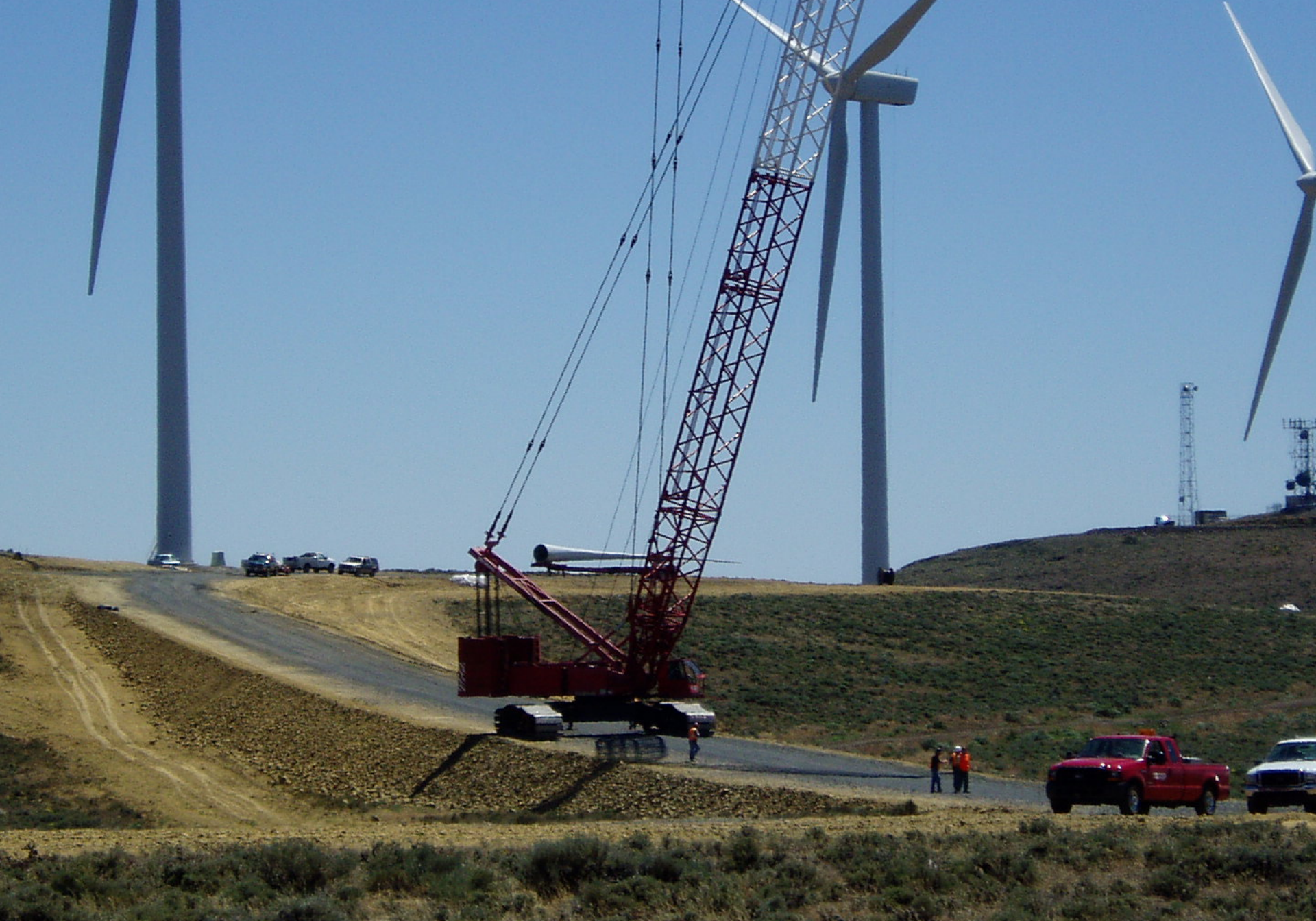
Road is 34 feet wide; Crane is 32.5 feet wide
