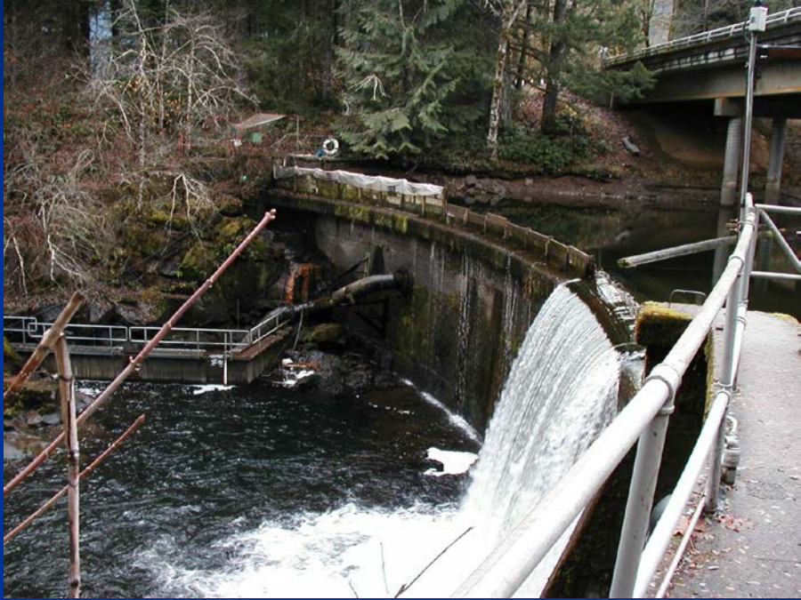
Hemlock Dam, Trout Creek Wind River Basin
