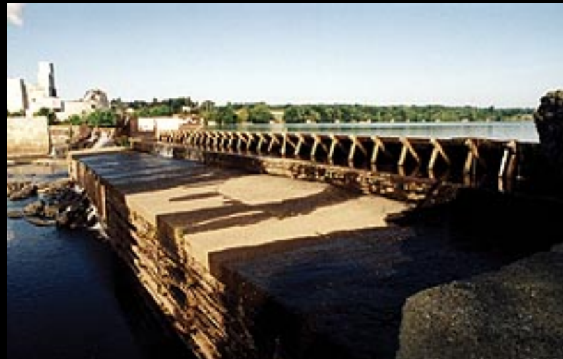
Greatworks Dam, Penobscot River
