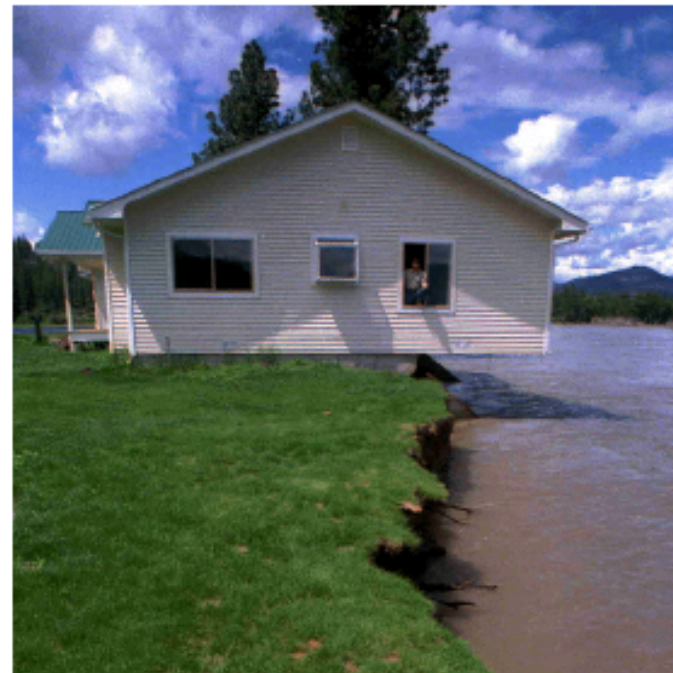
Figure 1-5. Riverine erosion can undercut structures
