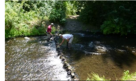
BTTF members remove a channel-spanning rock dam on the South Fork of Ahtanum Creek in 2015.
