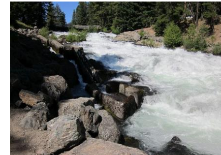
Clear Lake Spillway – No Functional Fish Passage Facilities
