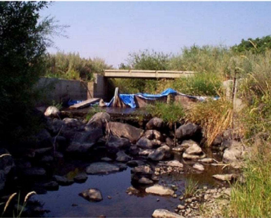
BEFORE: Irrigation dam blocks fish passage
