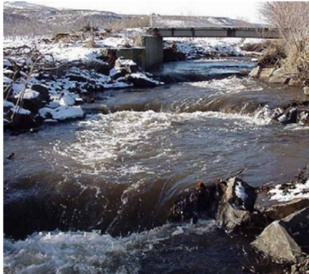
AFTER: Rock weirs allow full fish passage
