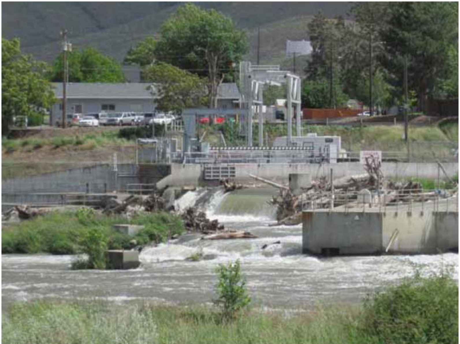
Figure 54. Prosser Dam with captured large woody debris (2010).
