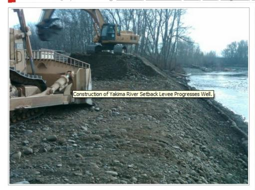
The Yakima River levee system is bustling with activity these days as the U.S. Army Corps of Engineers works to construct a setback levee measuring nearly 3,900 linear feet on the left bank of the Yakima River near Sportsman State Park.
