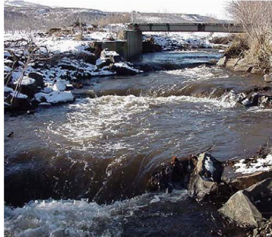
AFTER: Rock weirs allow full fish passage
