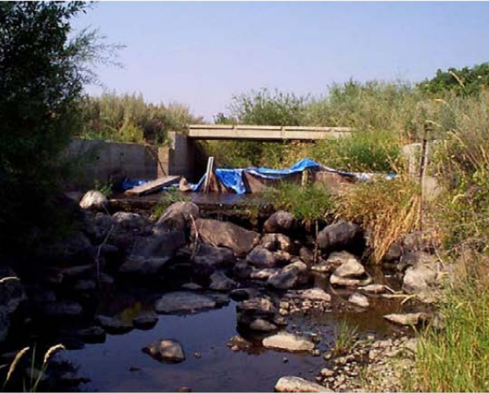
BEFORE: Irrigation dam blocks fish passage
