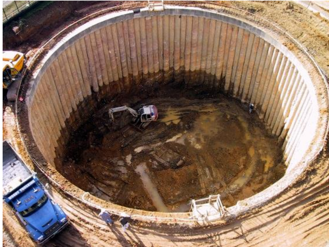
Secant Pile Example
