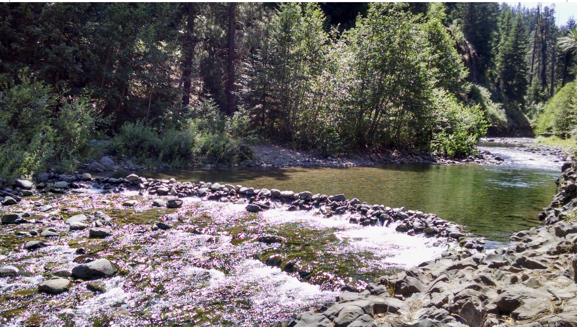
Recreation dam on Rattlesnake Creek
