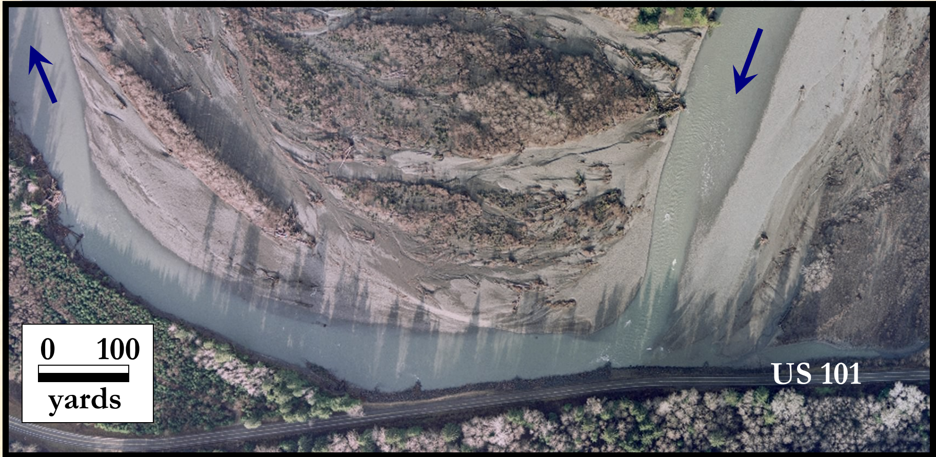
Hoh River project site in Spring of 2004 prior to construction.
