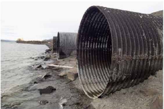
Site Photograph - culvert outlets
