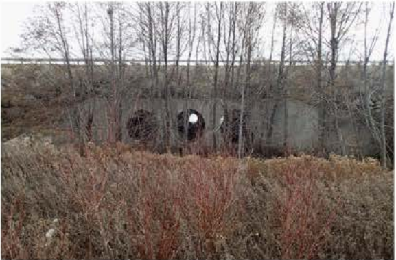
Site Photograph - culvert inlets
