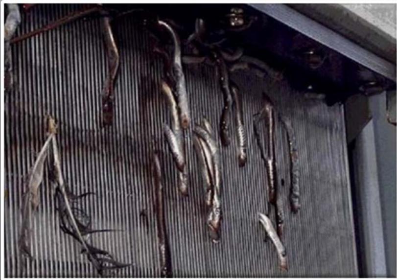
Juvenile lamprey impinged on turbine intake screen
