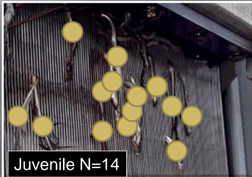
Juvenile lamprey impinged on turbine intake screen
