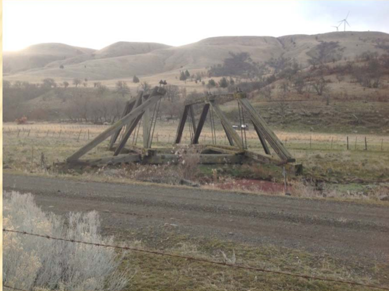
Bridge (left) that was washed off its piling foundation (right) by the 1964 flood.
