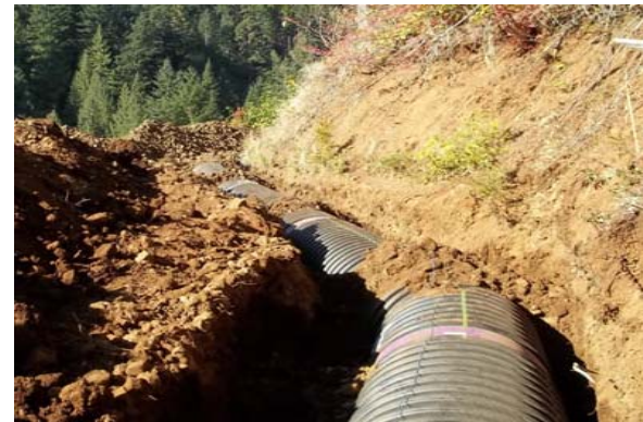
New pipe project
