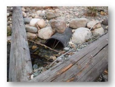
Performance of the infiltration gallery was not affected by the cobble/gravel deposits near the pipe outlet because the gallery invert is still well above the elevation of the deposited bed load. However it is recommended by the project engineer that the gravel/cobble mound be shoveled out by hand to recreate the post project plunge pool conditions and prevent additional sediment deposition from occurring at the pipe outlet.
