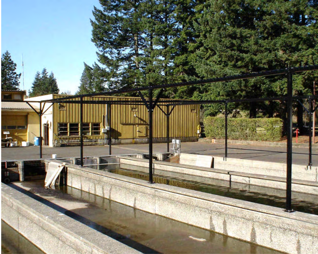
Figure 10. Cascade Raceways and Net Frame Photo (raceways 2,4,6 without overhead cover or predator nets in place)
