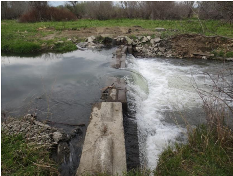
Figure 7. Unit 2 Diversion Dam in Toppenish Creek (river km 44.6), left channel looking downstream, a potential partial passage barrier for upstream migrating adult Pacific Lamprey.
