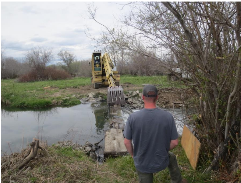
Figure 9. Toppenish Creek Unit 2 Diversion Dam (river km 44.6) left channel modification on April 7, 2015 (widening the thalweg width by increasing the gap between the ecology blocks in the center).
