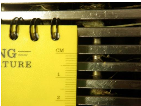
Figure G3-7. Bar screen mesh (screen in the lower part of the photo) has a 3.5~3.8 mm opening.
