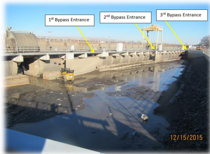
Photo G3. Overview of Chandler Diversion upstream of fish screens during the dewatered season.
