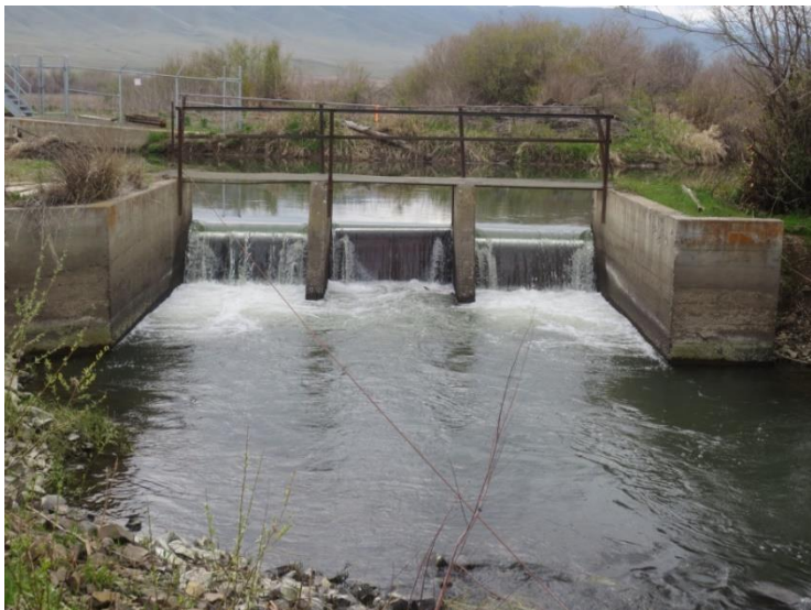
Figure E1-3. Unit 2 Diversion Dam in Toppenish Creek (river km 44.6), right bank looking downstream, a potential partial passage barrier for upstream migrating adult Pacific Lamprey.
