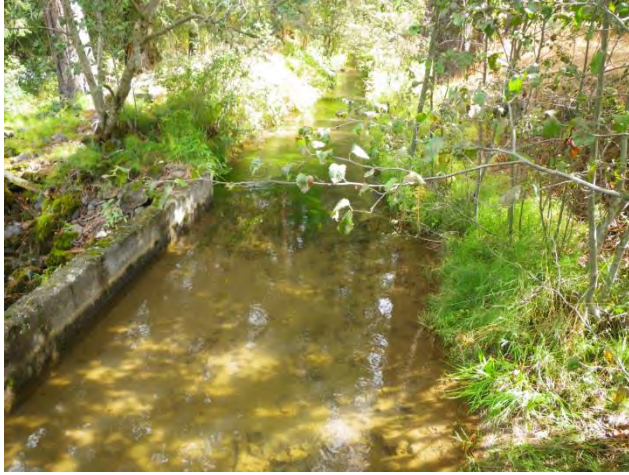
WS6: looking downstream in the diversion from the weir
