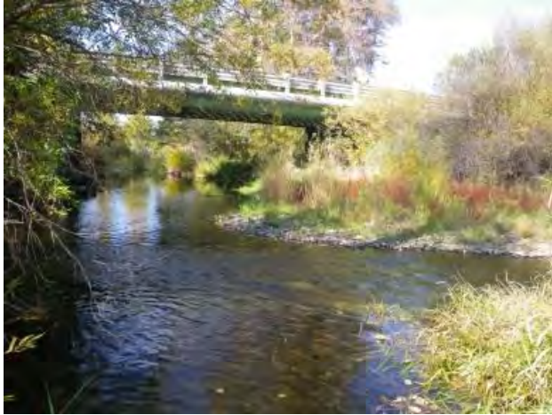
LK1: Looking downstream from survey area
