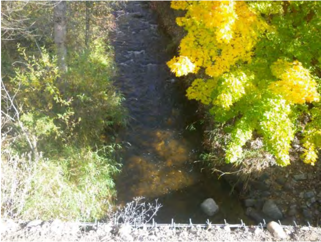
B-b (1): Upstream overview of marked site; channelized, and no available habitat observed (cobble and gravel only)
