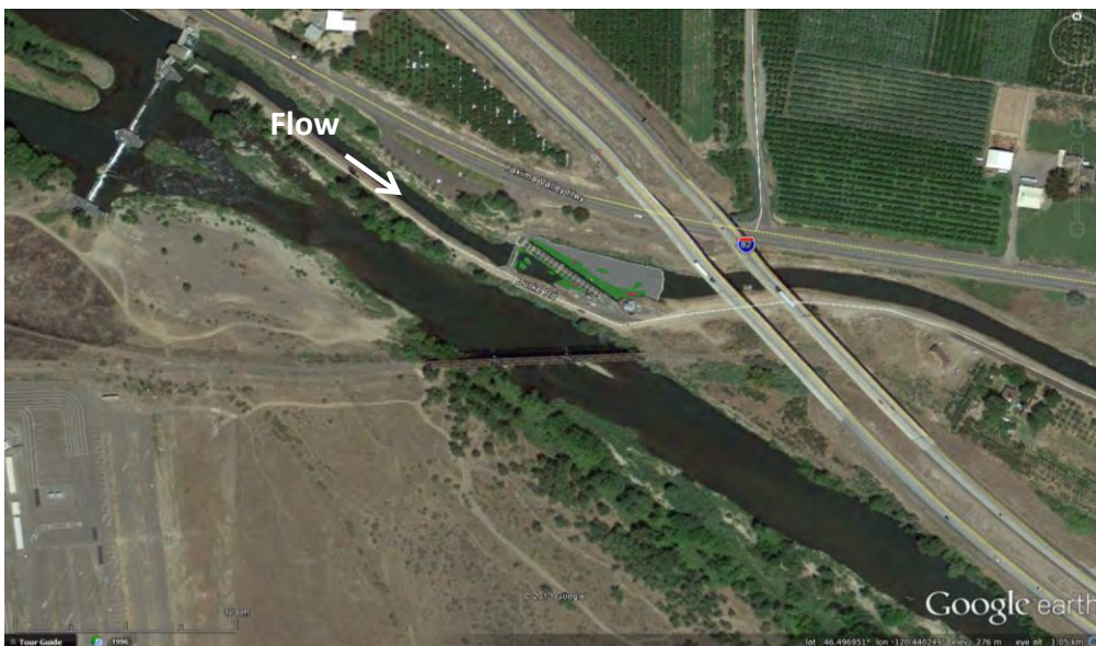
Photo 2a: Overview of Sunnyside Diversion.
