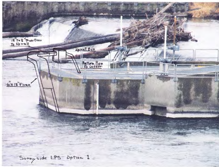
Figure 11. A photo with an engineer drawing depicting one of the routing options for an LPS structure at Sunnyside Dam (central ladder). This routing option would return lamprey to the central fish ladder, providing a short and easy access to enter the fish ladder. Preliminary radio telemetry results from USFWS indicate that many lamprey spent some time just downstream of the central fish ladder, and once lamprey entered and found the fish ladder, most fish were able to successfully pass the dam relatively quickly.
