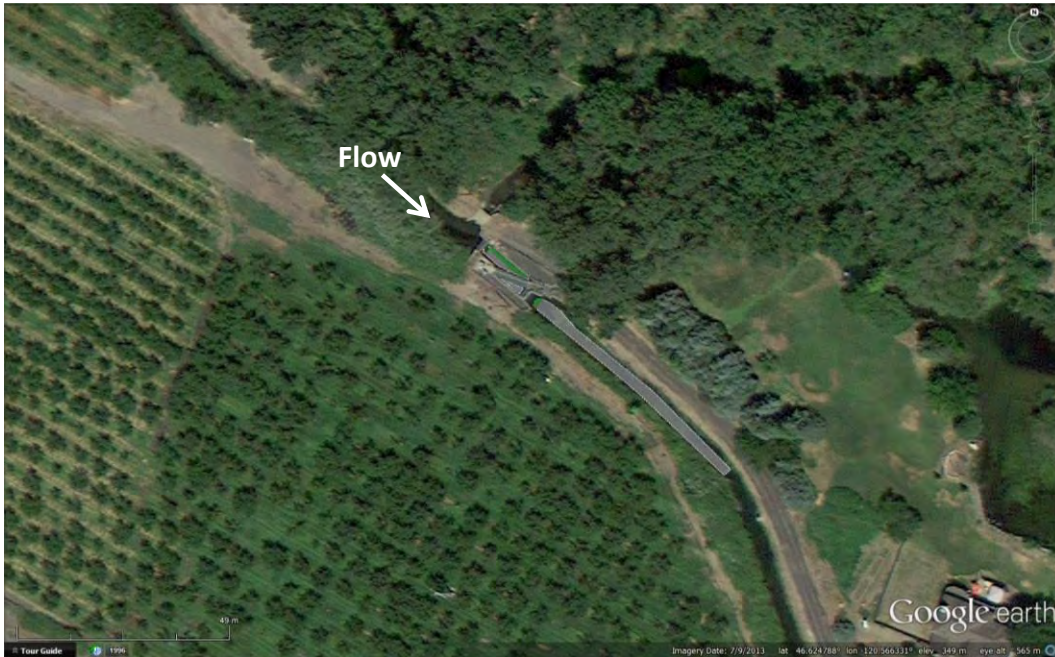
Photo 20a: Overview of Fruitvale Diversion.
