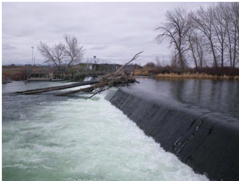
Sunnyside Dam Overview
