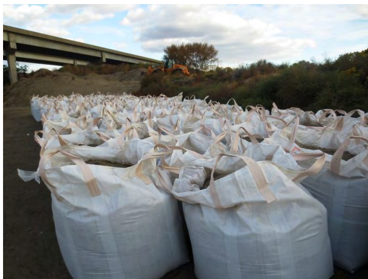
Photo F1: Hundreds of 1-ton sediment bags ready to be shipped off site at Sunnyside Diversion are indicative of the voluminous amount of fine sediment collected behind the fish screens there.
