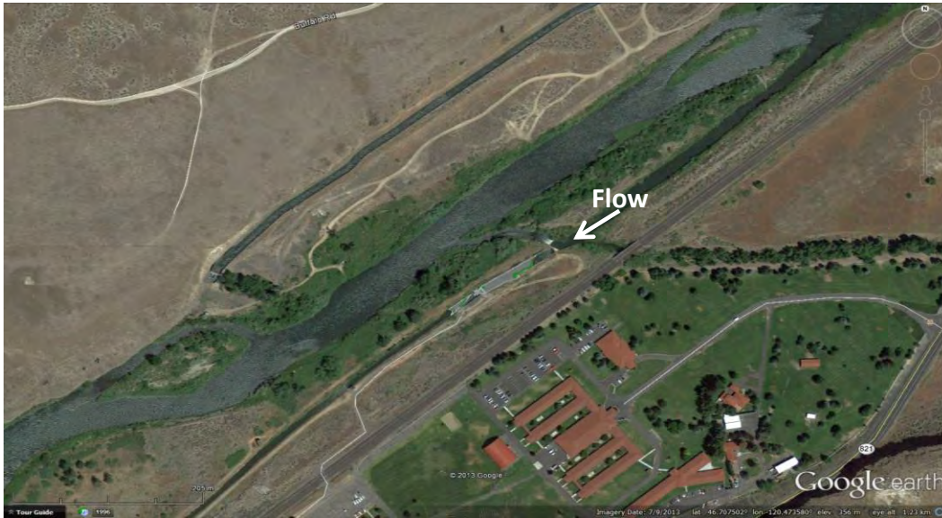
Photo 6a: Overview of Selah-Moxee Diversion.
