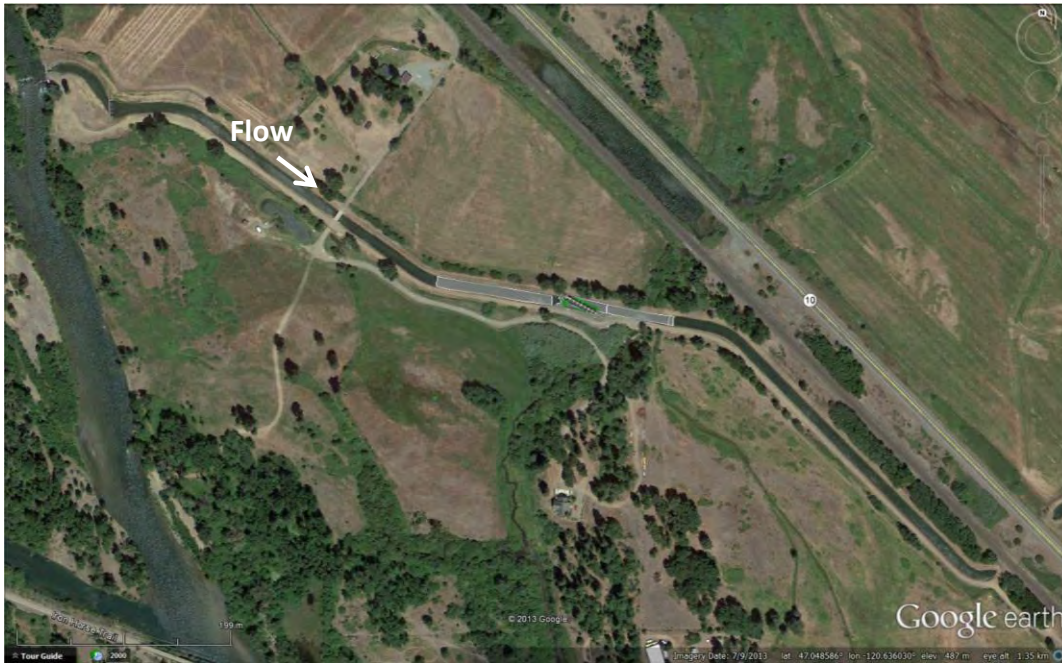
Photo 8a: Overview of New Cascade Diversion.
