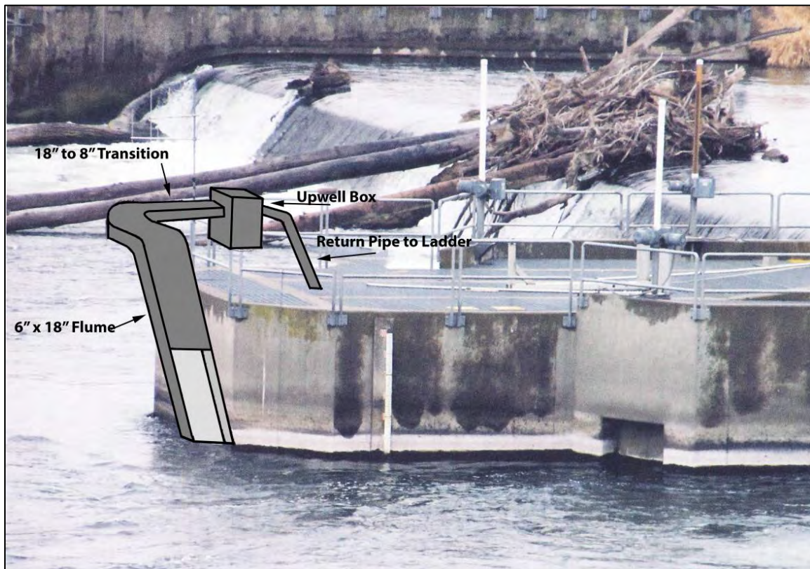
Figure 25. Photograph of the center fishway at Sunnyside Dam with concept drawing of LPS that returns lamprey into the fish ladder (J. Simonson, Fishhead Technology and Mark Nelson USFWS).
