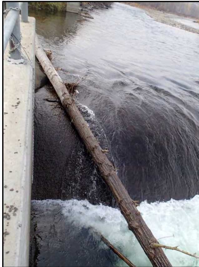
Figure 23. Photograph of the right bank of Cowiche Dam showing a log hung up on crest that deflects flow and calms turbulence at the intersection of the dam face and fishway wall, resulting in conditions that may favor lamprey climbing behavior to pass a dam.
