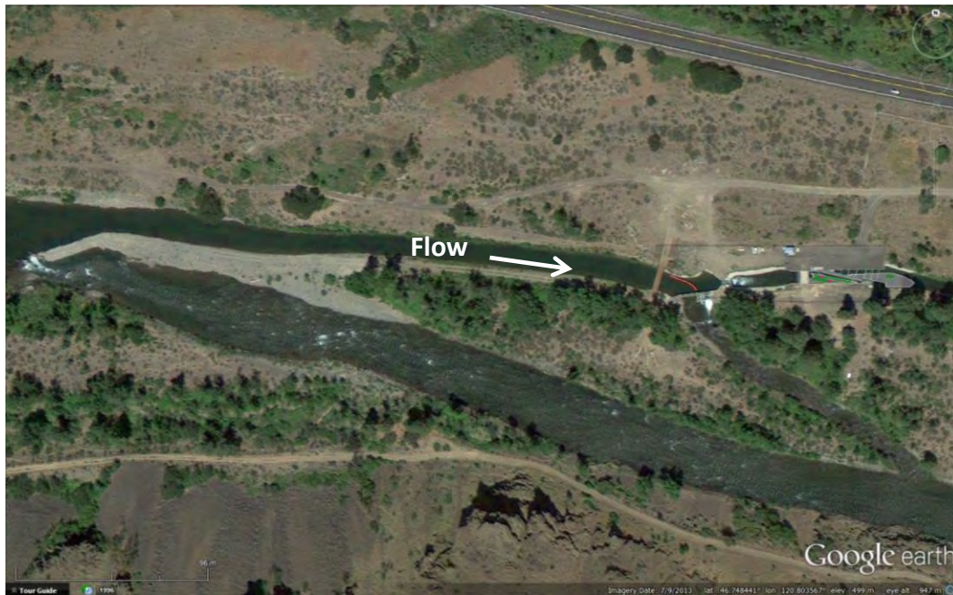
Photo 19a: Overview of Naches-Selah Diversion.
