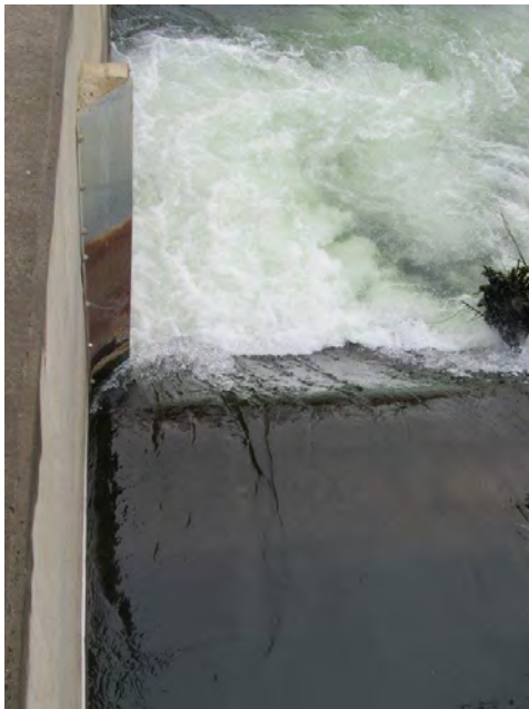
Figure 14. A photo showing the existing deflector placed just downstream of the dam. If a deflector was placed upstream of the dam (as shown in Figure 9), it may be able to create a gentler flow on the spillway where lamprey could potentially pass.
