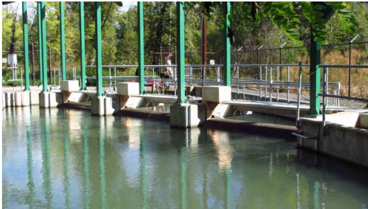
Figure 2. Looking upstream towards the three rotary drum fish screens at Congdon Diversion.
