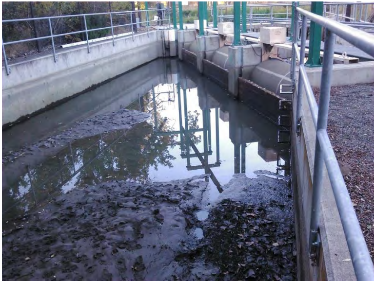
Figure 20. Congdon Diversion after dewatering (looking upstream towards the three rotary drum fish screens). An abundance of fine sediment and organic matter is available downstream of the screens.
