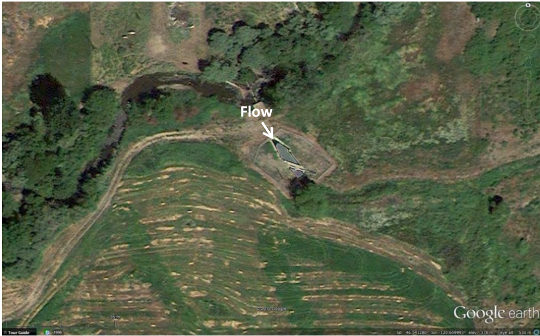
Photo 12a: Overview of Lower WIP Diversion
