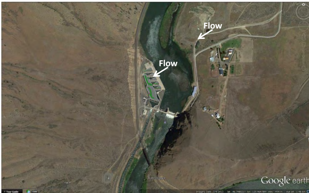
Photo 7a: Overview of Roza Diversion.
