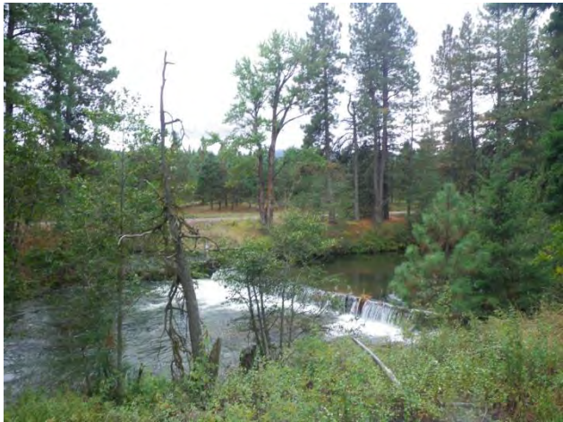
WS6: View from left bank of diversion weir
