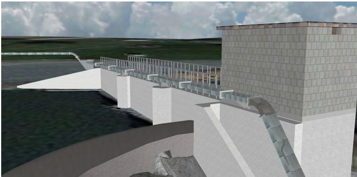
Figure 16. The second section for the proposed LPS on the left bank at Prosser Dam, showing the flume extending across the Chandler Diversion headgate.
