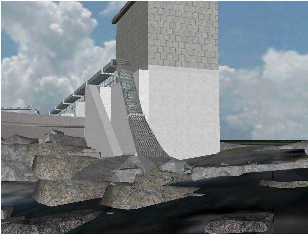
Figure 20. An alternative view of the entrance to the proposed LPS on the left bank at Prosser Dam.
