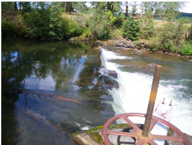
WS6: View from right bank of diversion weir and the head gate
