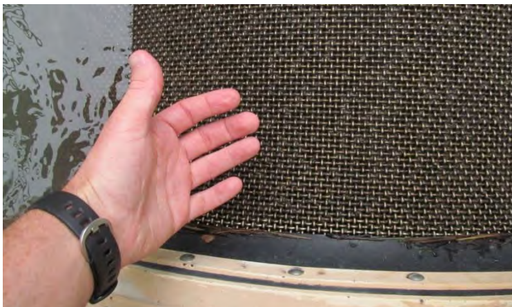
Figure 3. Woven wire mesh with a 3/32" (2.84 mm) opening at Congdon Diversion.
