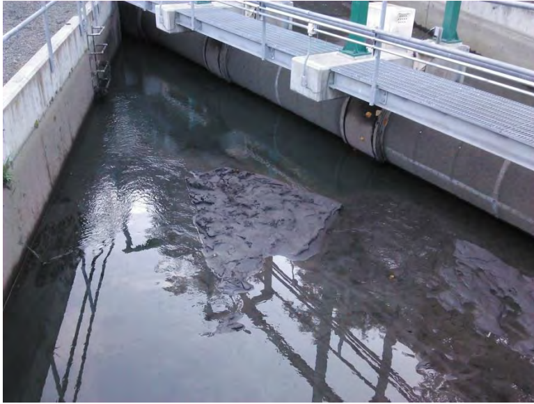
Figure 19. Congdon Diversion after dewatering (looking downstream towards the three rotary drum fish screens). An abundance of fine sediment and organic matter is available upstream of the screens.
