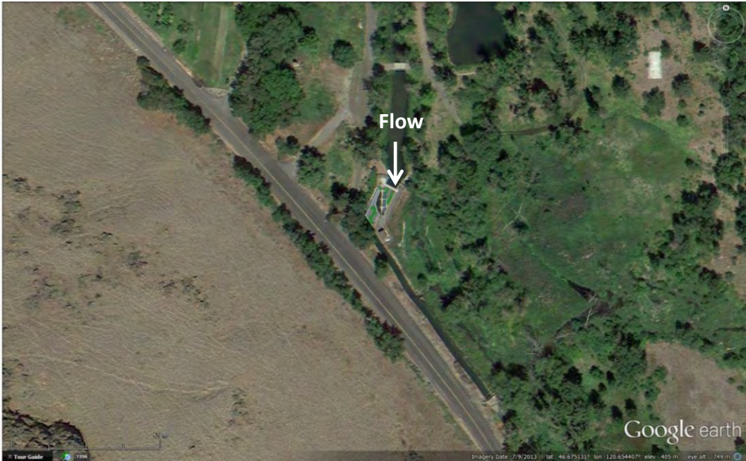
Photo 16a: Overview of Congdon Diversion.
