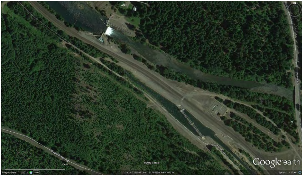
Figure 11: Overview of Kittitas-Easton Diversion
