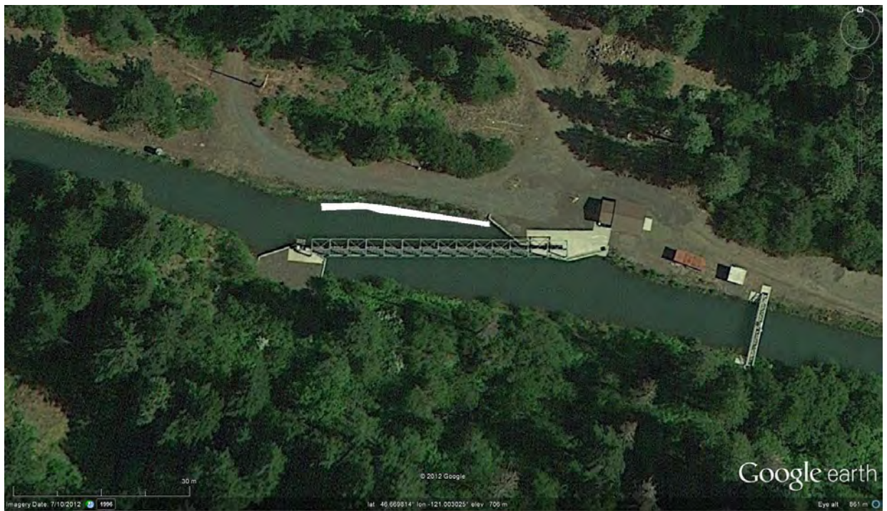
Figure 4: Close up of Yakima-Tieton Screens
