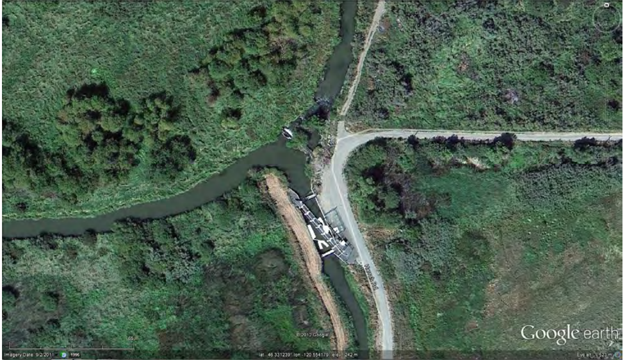
Figure 31: Overview of Unit 2 Feeder Diversion
