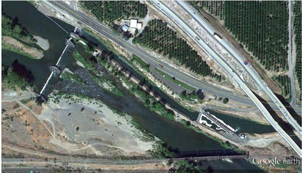
Figure 27: Overview of Sunnyside Diversion
