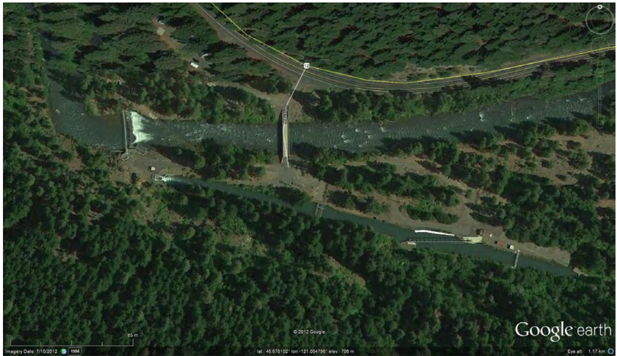
Figure 3: Overview of Yakima-Tieton Diversion
