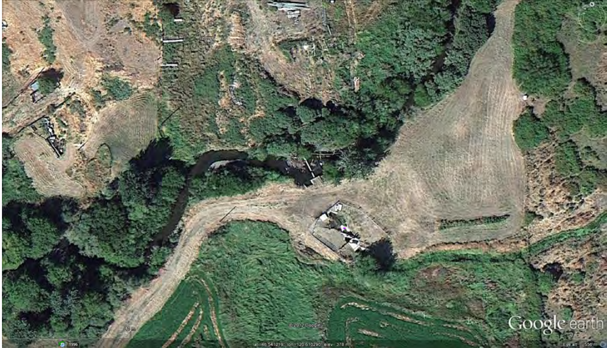
Figure 17: Overview of Lower WIP Diversion
