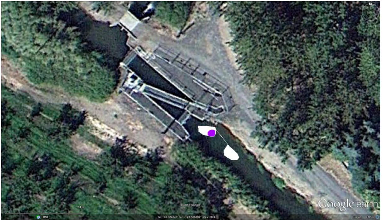
Figure 8: Close up of Cowiche Screens
