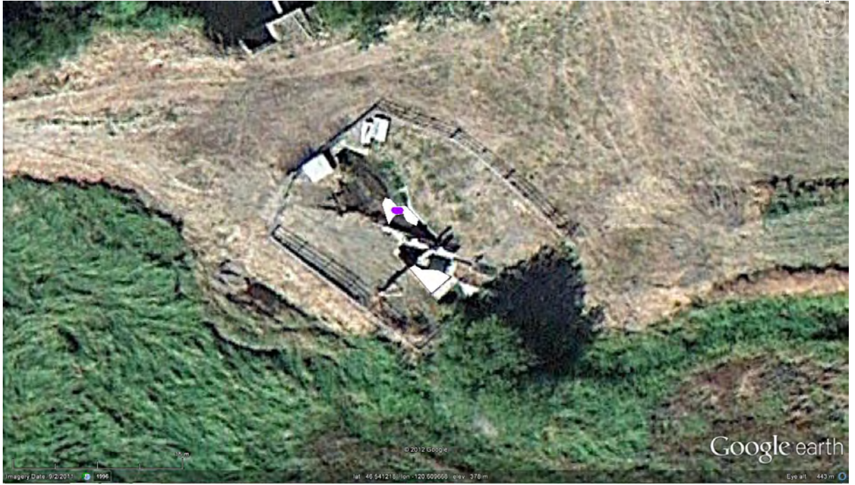
Figure 18: Close up of Lower WIP Screens
