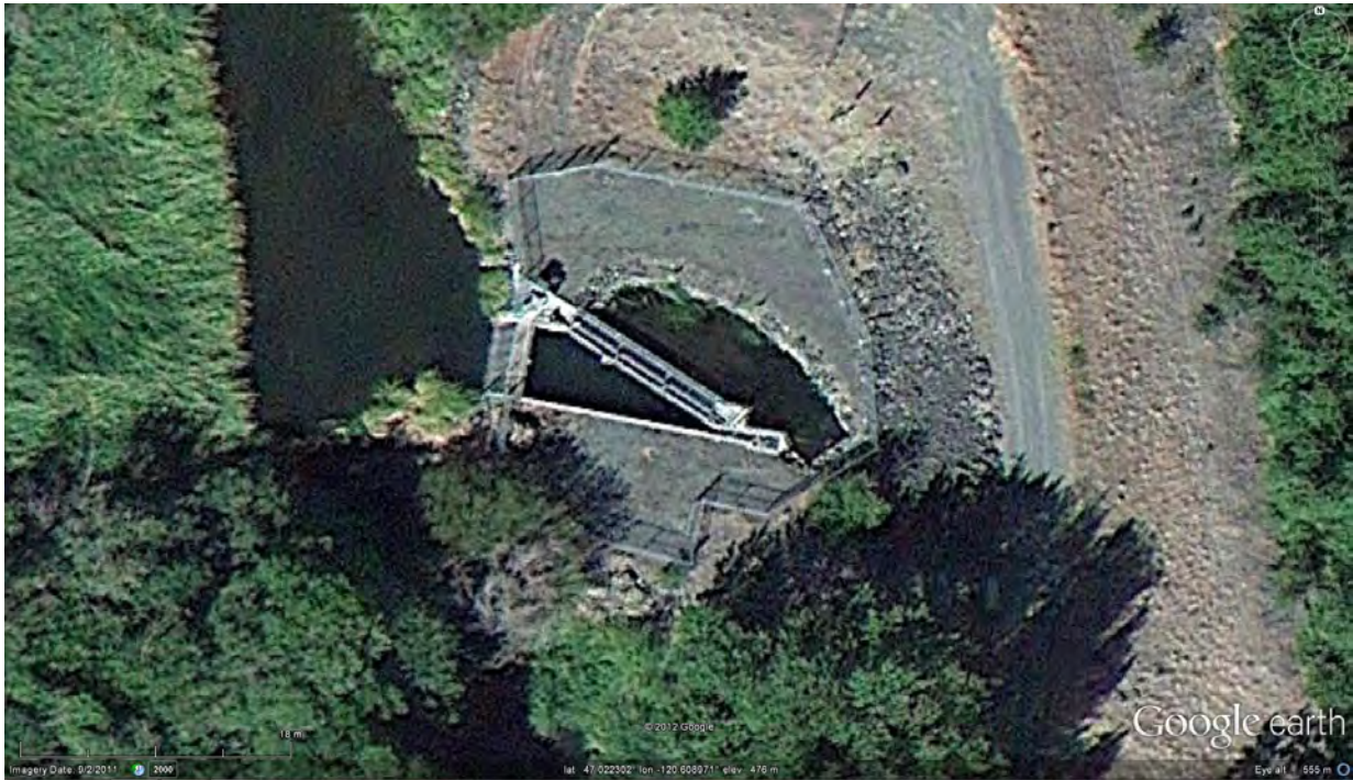
Figure 16: Close up of Ellensburg Mill Screens
