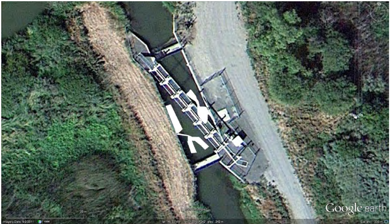
Figure 32: Close up of Unit 2 Feeder Screens
