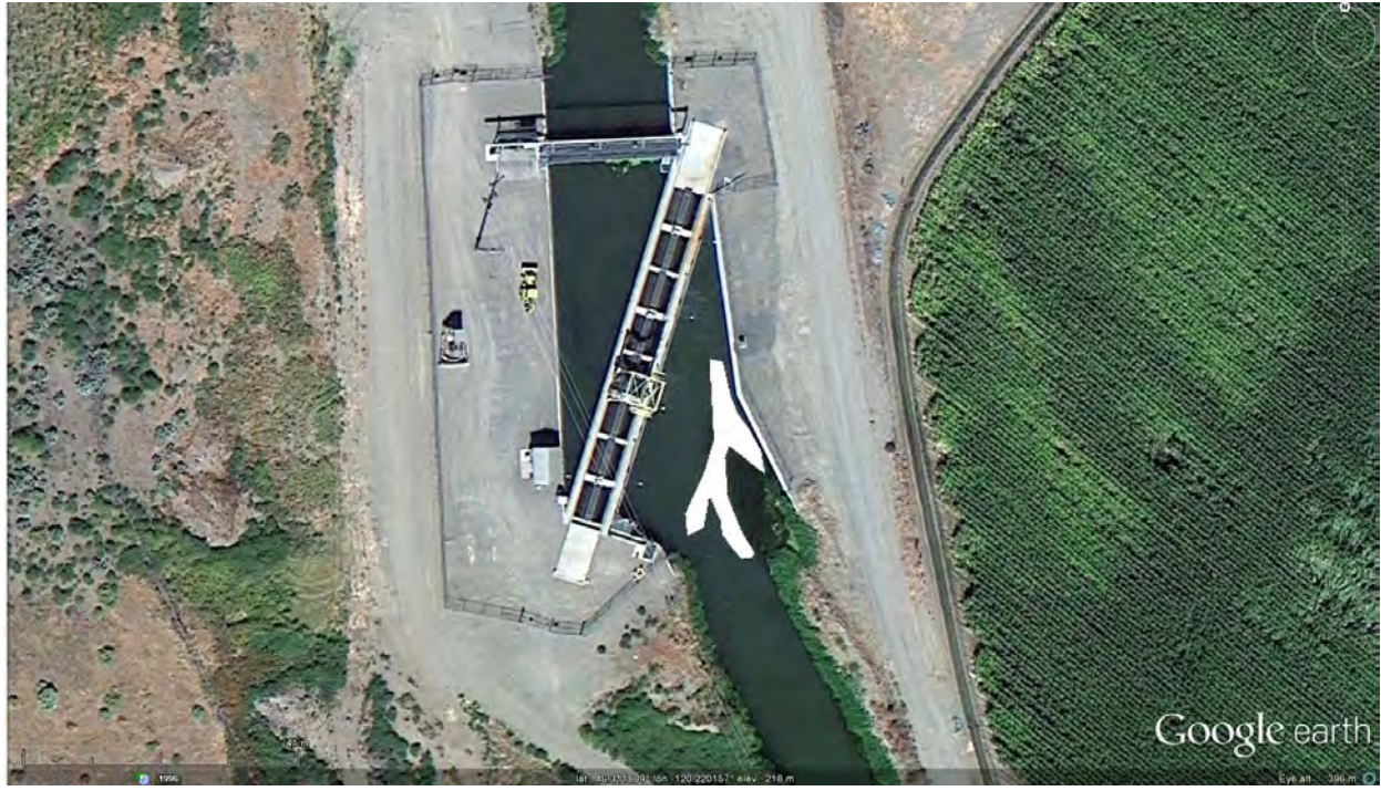
Figure 30: Close up of Toppenish-Satus Screens
