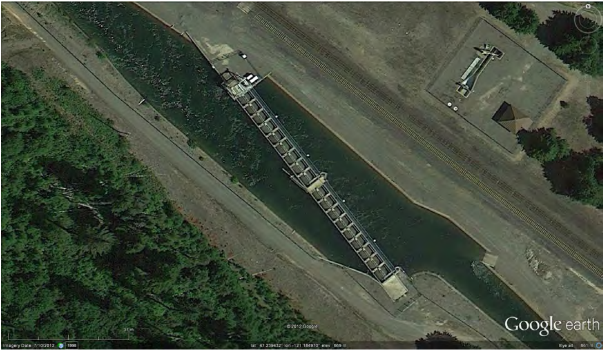
Figure 12: Close up of Kittitas-Easton Screens
