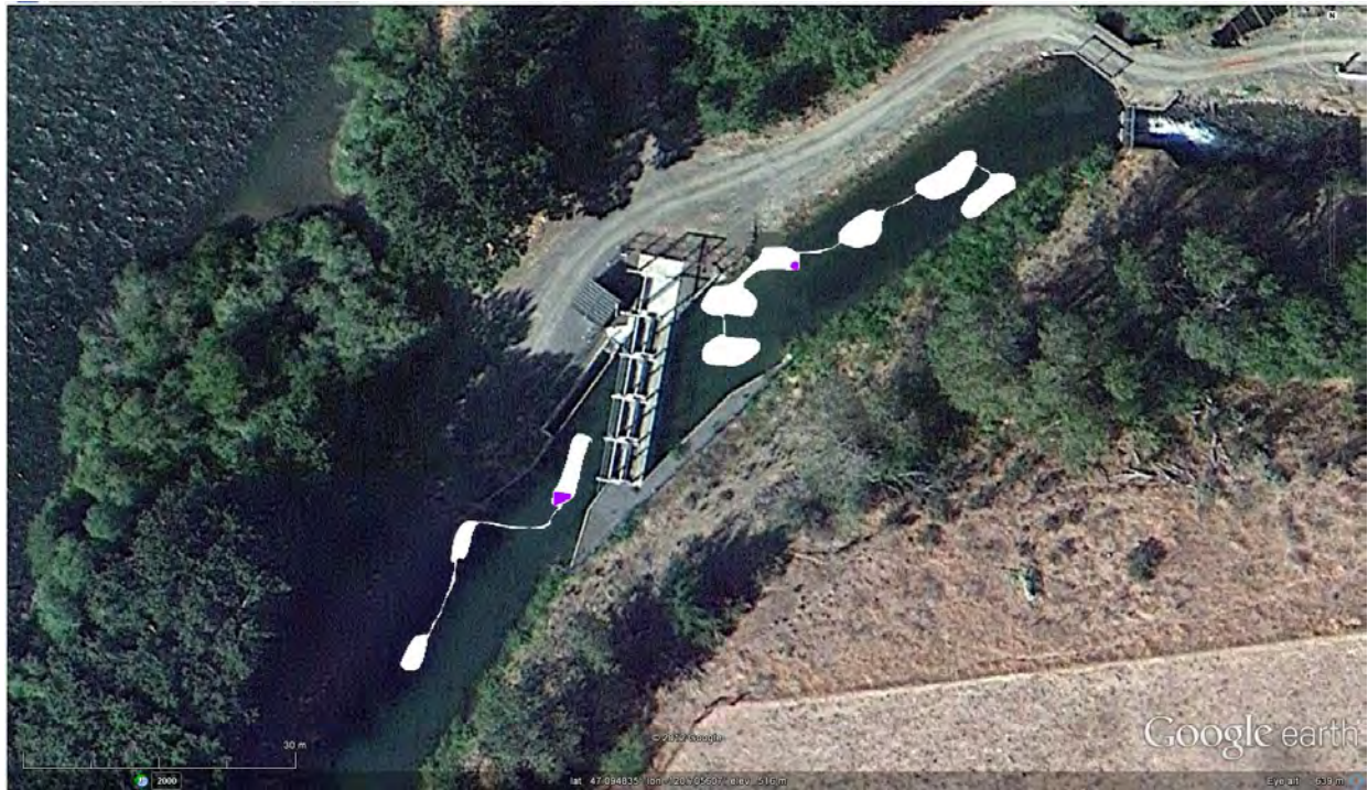
Figure 6: Close up of Westside Screens
