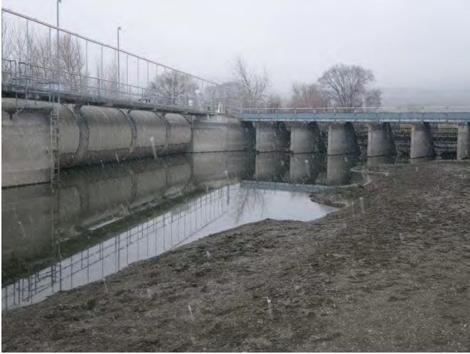
11/28/12: View of the screens, trash racks, and muddy bank during the survey in snow.
