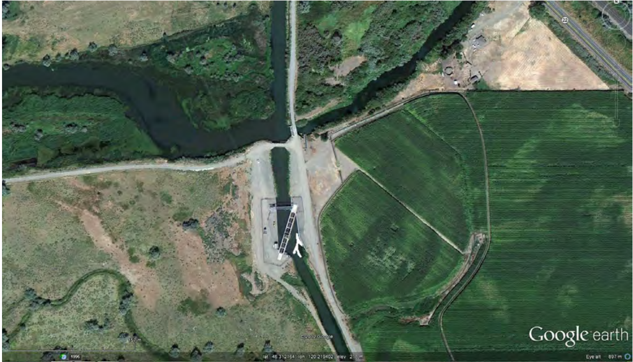
Figure 29: Overview of Toppenish-Satus Diversion
