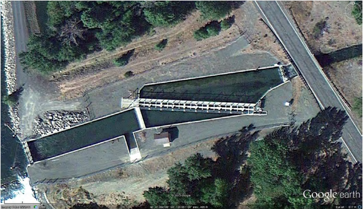
Figure 26: Close up of C-Town Screens
