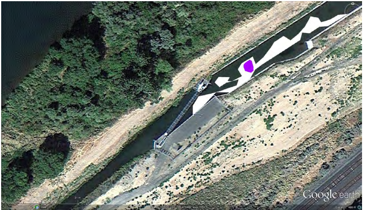
Figure 22: Close up of Selah-Moxee Screens
