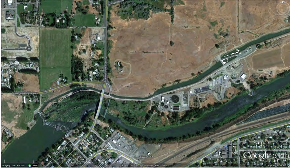
Figure 23: Overview of Chandler Diversion
