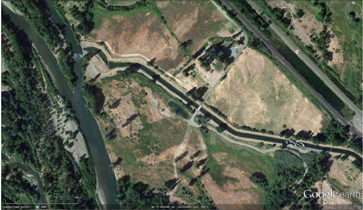
Figure 13: Overview of New Cascade Diversion
