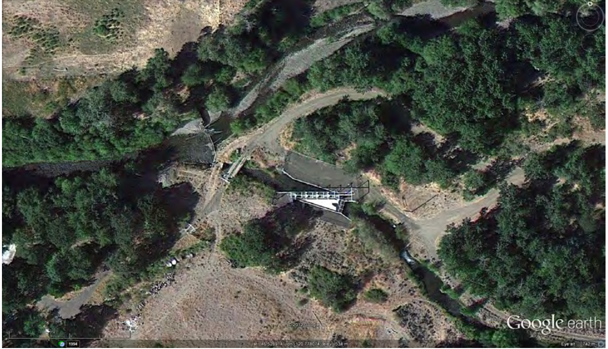
Figure 19: Overview of Upper WIP Diversion
