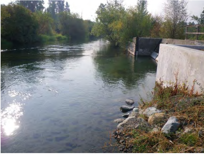
Dryden Canal: very little amounts of silt along bank mixed with gravel
