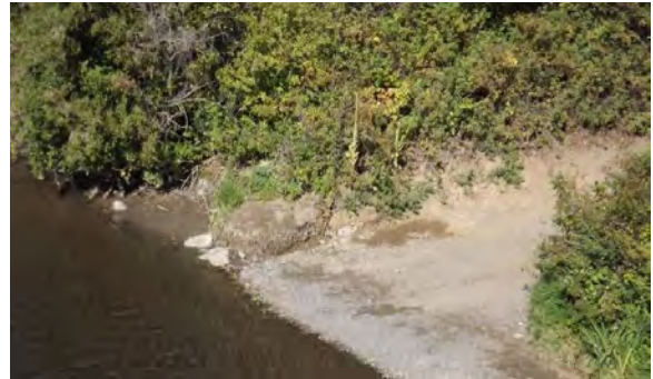
Figure 15. View of boat launch from the foot bridge. Sediment primarily present on upstream side of boat launch.
