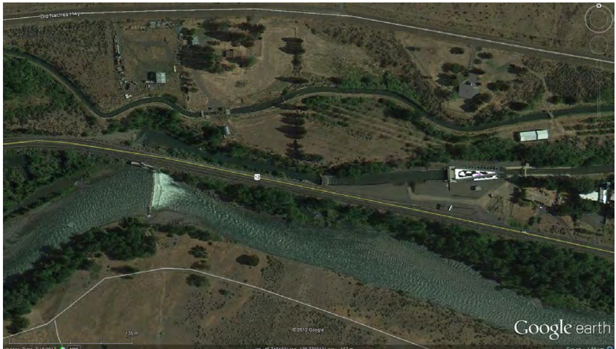
Figure 37: Overview of Wapatox Diversion
