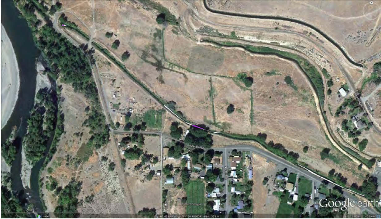
Figure 9: Overview of Union Gap Diversion
