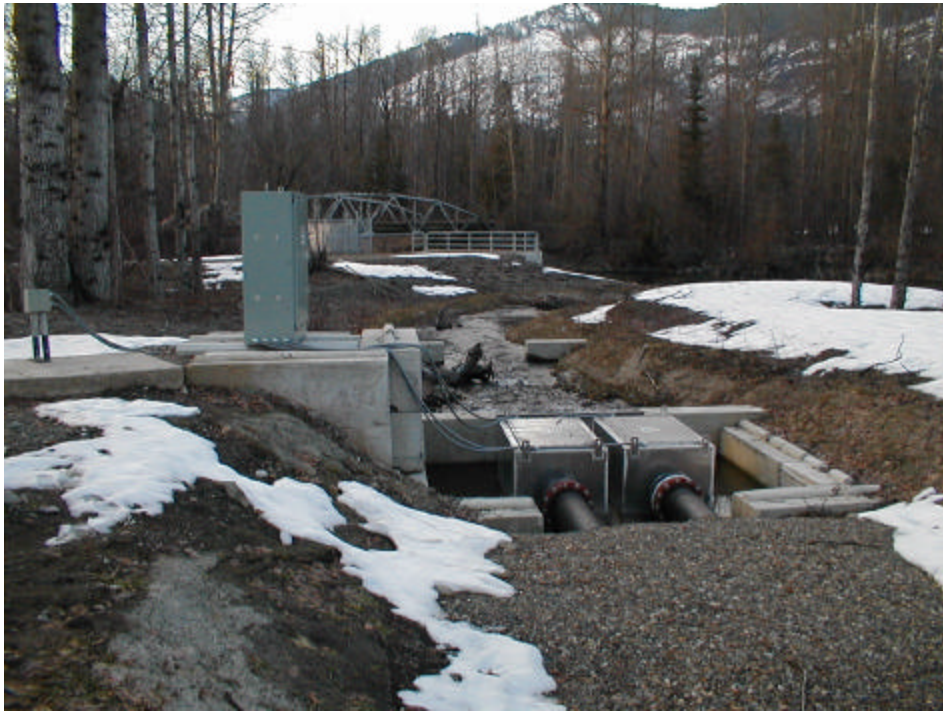
Figure 5. This photograph shows the Easton acclimation site discharge pipes and PIT-Tag detection system that are similar at all three acclimation sites.
