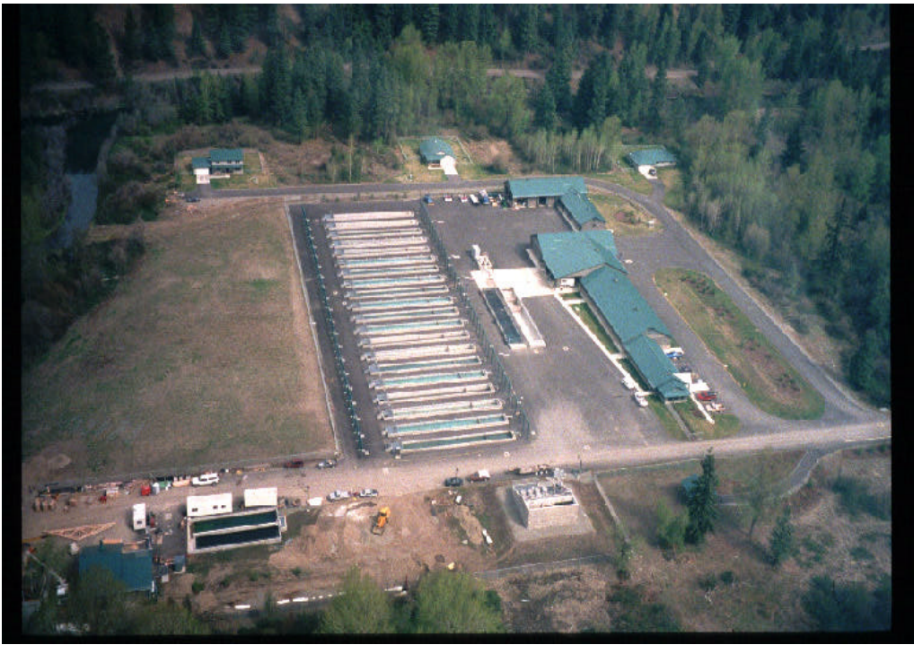
Figure 9. This photograph shows an aerial view of Cle Elum Supplementation and Research facilities.
