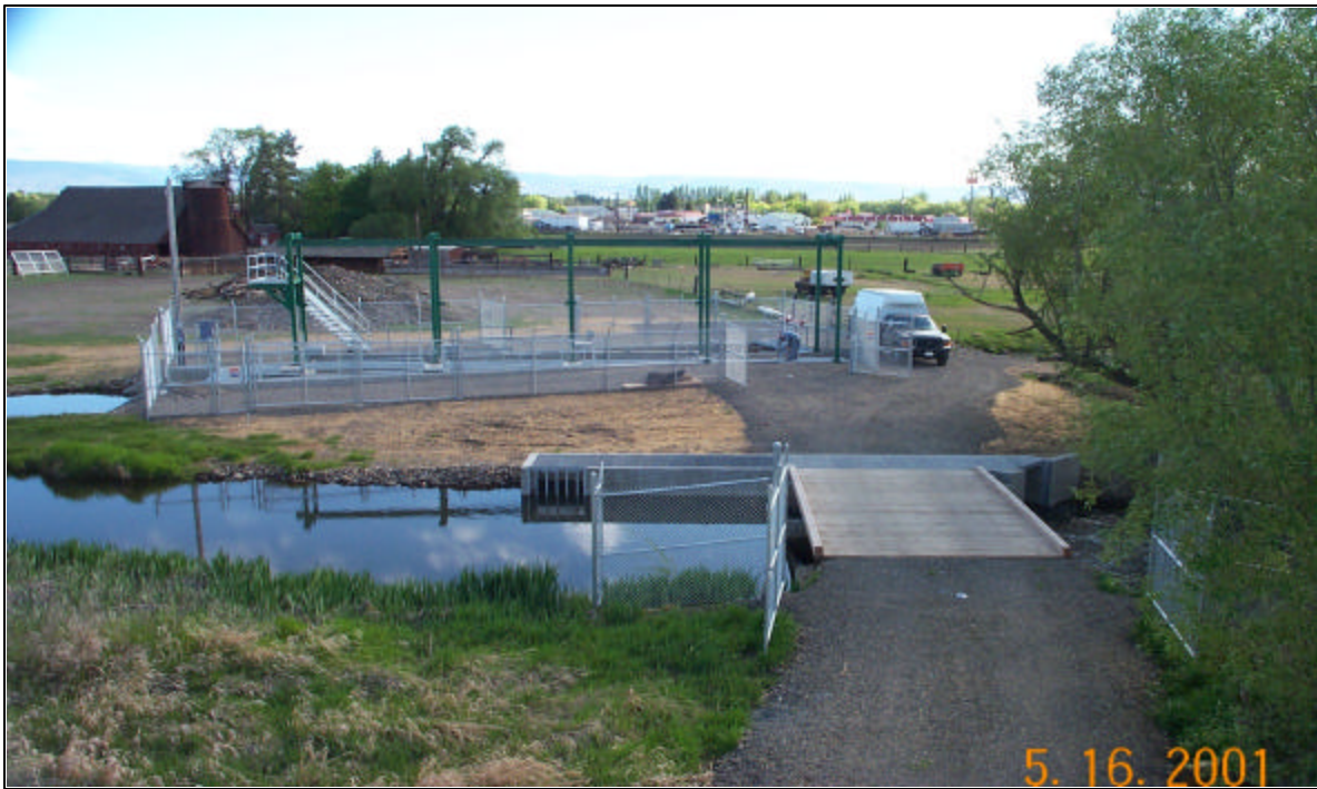
Figure 15. Newly completed fishway on Wilson Creek (rivermile 8).
