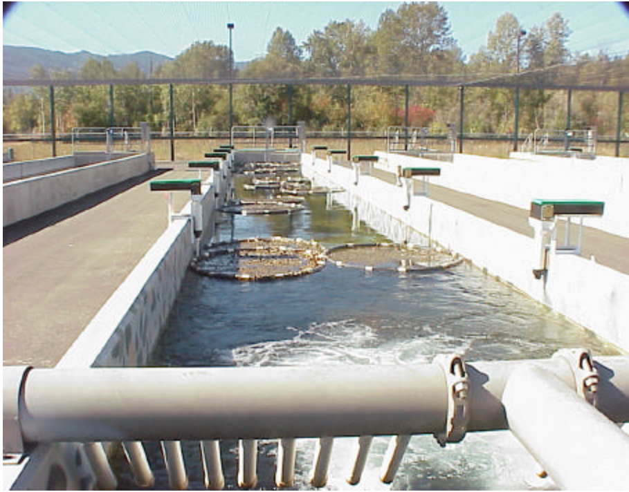
Figure 1. This photograph shows one of the semi-natural treatment (SNT) raceways at the Cle Elum Hatchery. Each SNT raceway has camouflaged painted raceway walls, shade covers, instream cover (Christmas trees), and underwater feeders.
