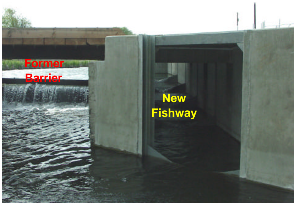
Figure 16. Bull Ditch Screen and Ladder at Wilson Creek. Constructed during the winter of 2000-01 at a cost of approximately $565,000.
