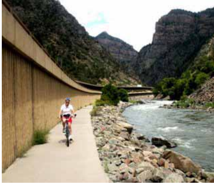
Figure 3 - A view of I-70 through Glenwood Canyon, Colorado. The roadway is elevated above the floodplain, bifurcated on separate levels, stepping up the hillslope with a retaining wall and on a viaduct structure. There is a multiple use trail separated from the travel lanes. The concrete retaining wall bears a form line color and texture, and could easily be made to look more like the natural stone.
