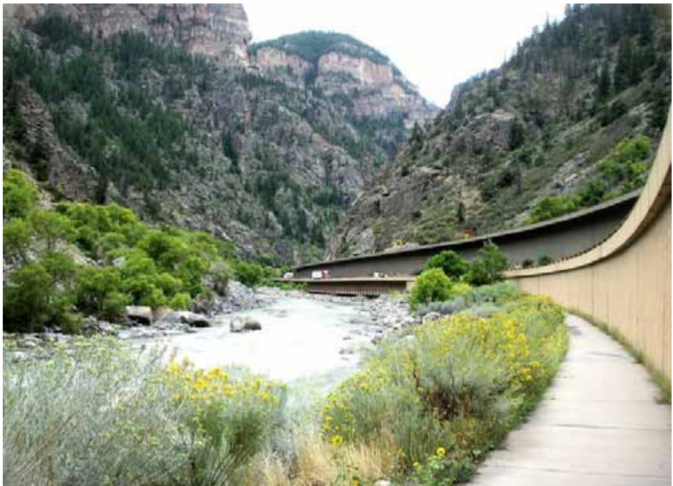
Figure 2 - I-70 through Glenwood Canyon, Colorado. The roadway is elevated above the floodplain, bifurcated on separate levels, stepping up the hillslope with a retaining wall and on a viaduct structure. There is a multiple use trail separated from the travel lanes. The retaining wall could bear a form line color and texture more like the natural stone.
