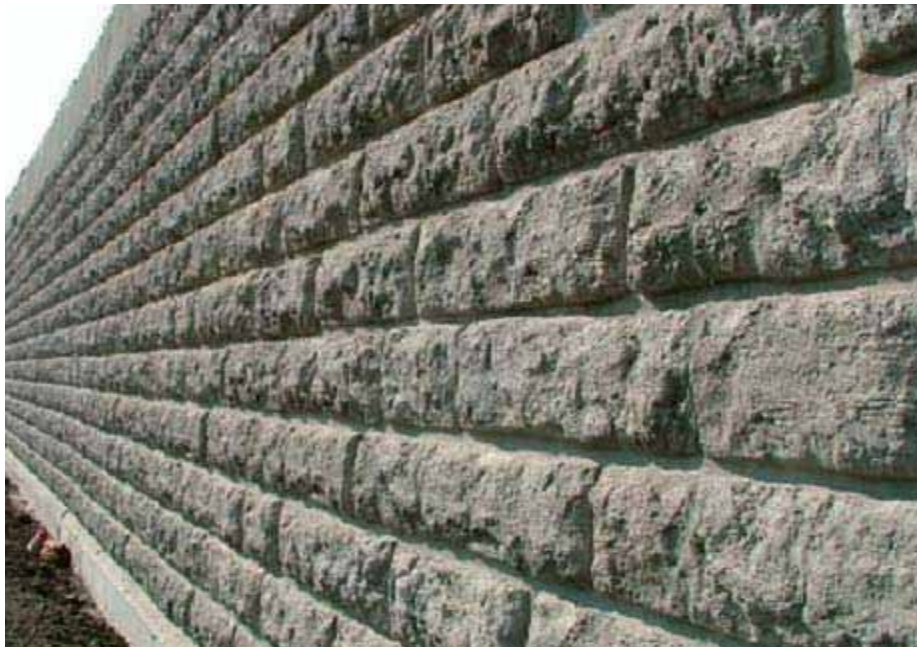
Figure 4 - Any of the project's retaining walls could bear a form line color and texture more like the natural stone finish, color and texture shown in this example. The texture is a large, coarse stone block, in regular courses. The color mimics the native stone nearby.
