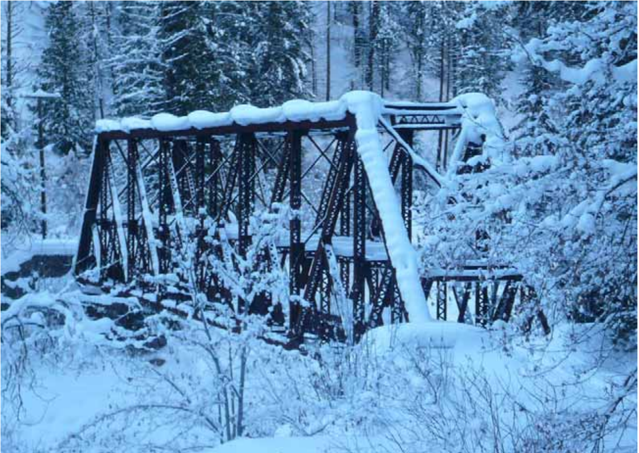
Figure 7-1. Penstock Bridge in the Project Reach
