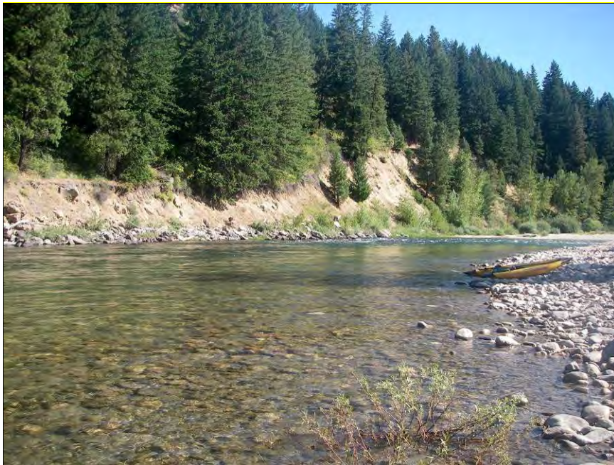
Figure 52. Erosion along the right bank continues upstream at this meander bend near RM 39.25.
