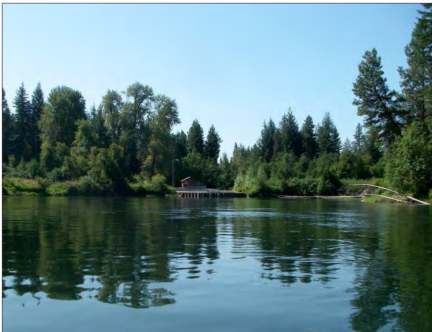
Figure 93. Small concrete retaining wall at meander bend just upstream from the WDFW hatchery facility (August 2011).
