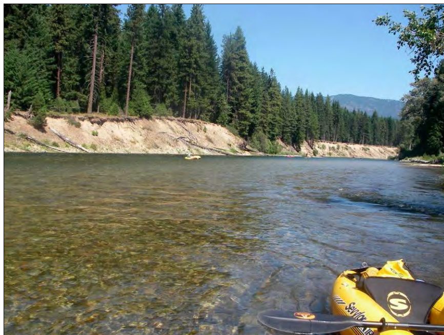
Figure 128. Bank erosion was primarily associated with moderately steep bank terraces along Reach 10 on river-left (August 2011).
