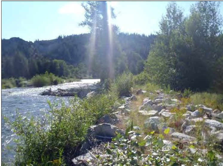
Figure 44. Riprap on river-right (RM 42.8).
