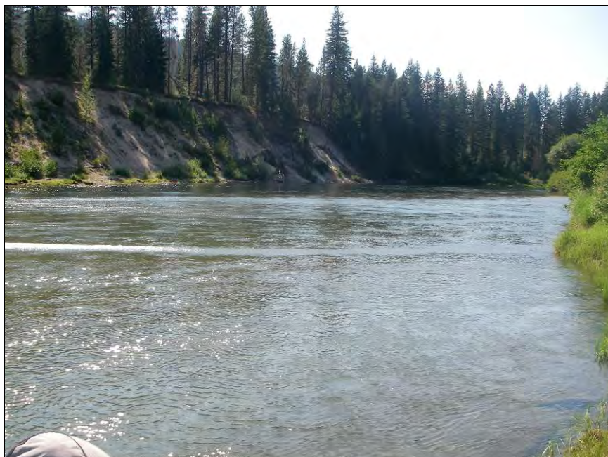
Figure 112. Bank instability was observed along many of the steep terrace banks throughout Reach 9 (August 2011).
