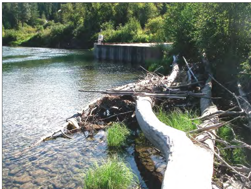
Figure 100. Concrete intake structure at the WDFW hatchery facility (August 2011).
