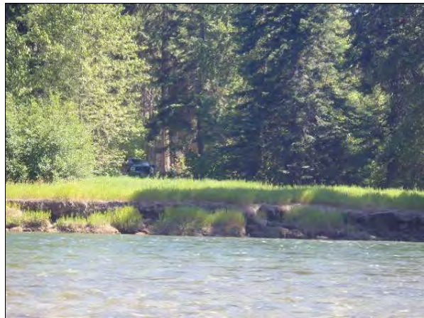
Figure 76. Left bank slumping due to lack of riparian vegetation.
