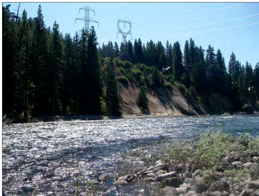
Figure 74. Transmission line clearing affects the riparian buffer and erosion near RM 44.45 (August 2011).
