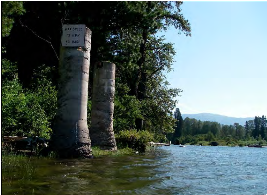
Figure 139. Remnant concrete pilings on river-left, Reach 11 (August 2011).
