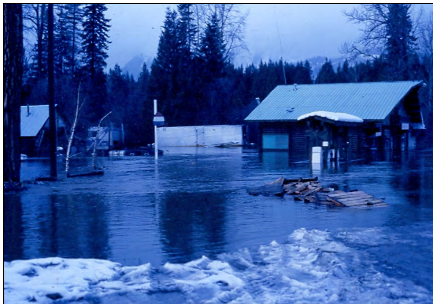
Figure 20. Flooding at the Headwaters Tavern near the upstream end of the study area. Photo date unknown (assumed Nov, 1990) (Photo courtesy of Bryon Newell).
