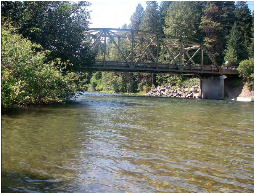
Figure 116. Bank armoring and channel confinement near the Hwy 207 Bridge, Reach 10 (August 2011).
