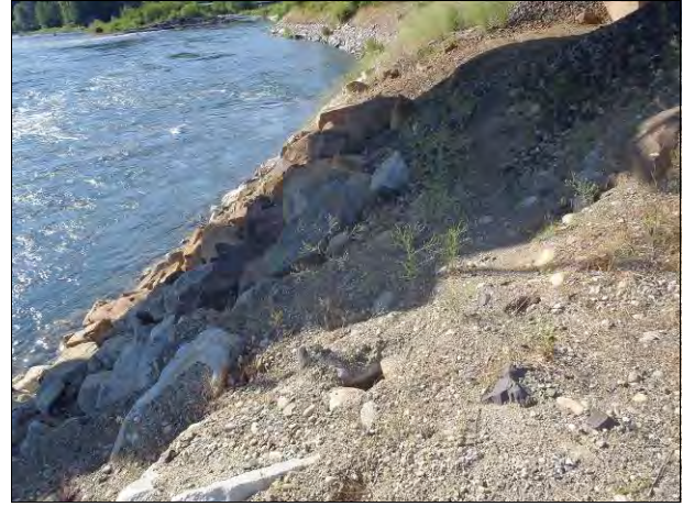
Figure 53. Right bank armoring
