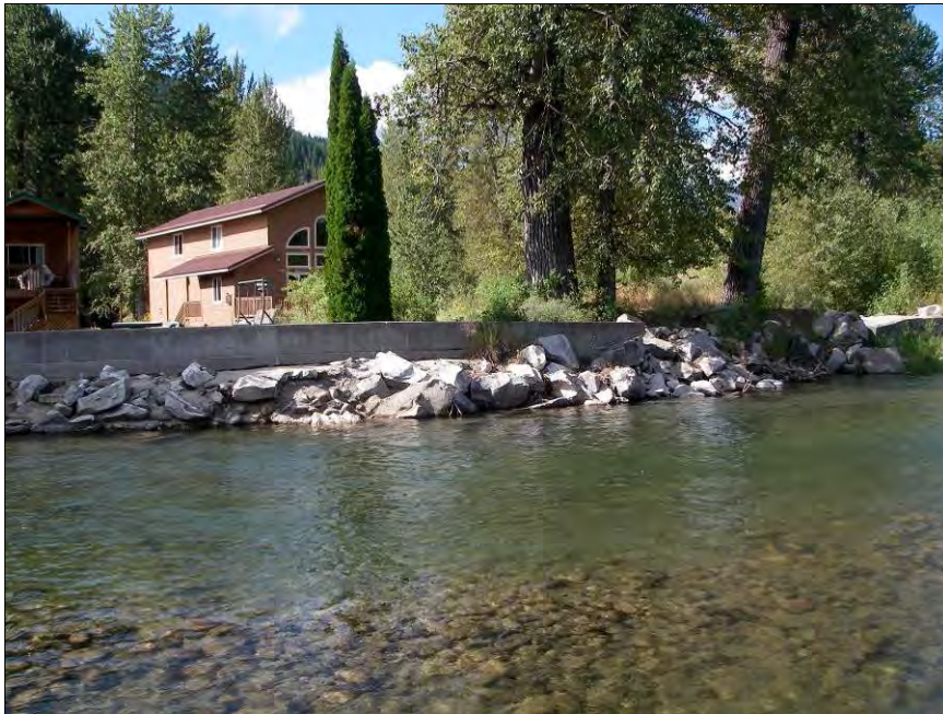
Figure 51. Concrete bank armor and riprap prevent natural channel process along much of Reach 3’s right bank as seen near RM 41.7 (August 2011).
