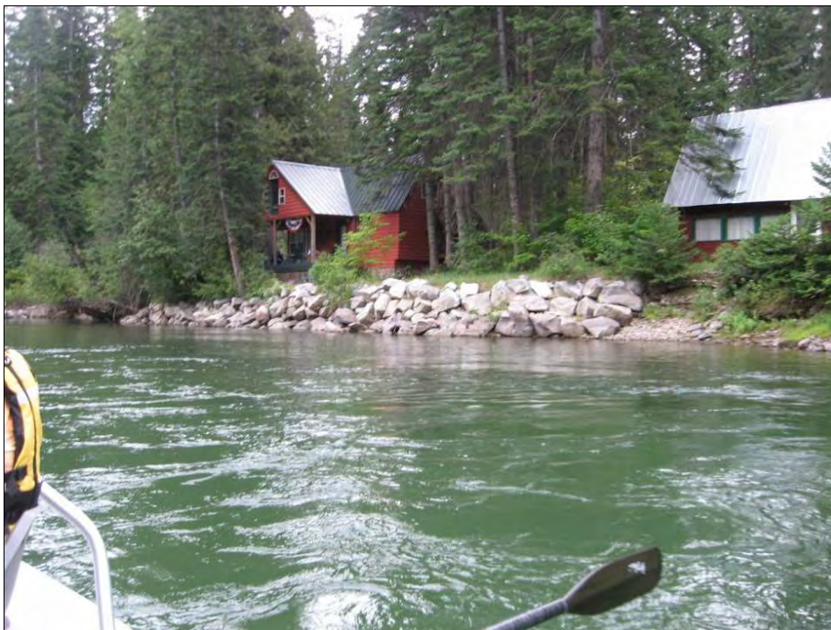
Figure 17. Residential development and bank hardening near the upstream end of the study area.
