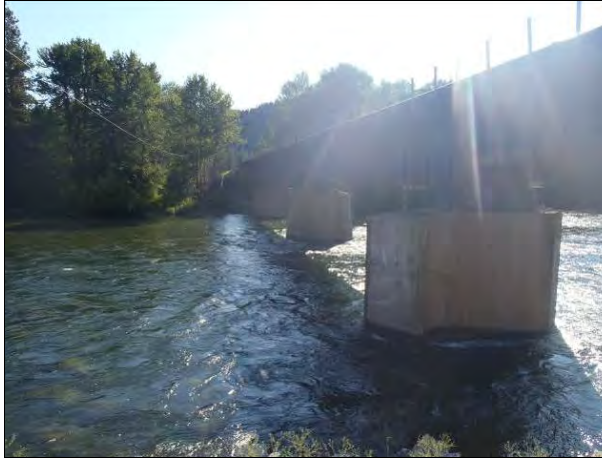
Figure 52. Burlington Northern Railroad Bridge Pilings
