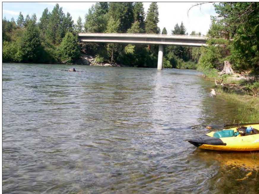
Figure 73. Beaver Valley Rd Bridge bisects the upper portion of Reach 5, where the channel is artificially confined by riprap armoring (August 2011).
