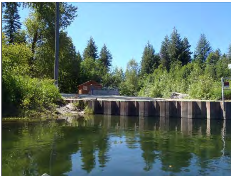
Figure 82. WDFW Chiwawa Ponds Fish Hatchery intake structure.
