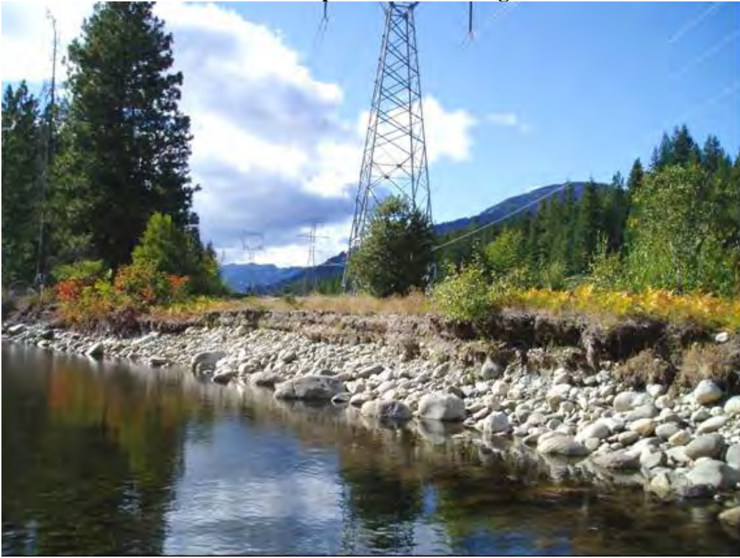
Bank erosion from power line crossing at RM 6.2
