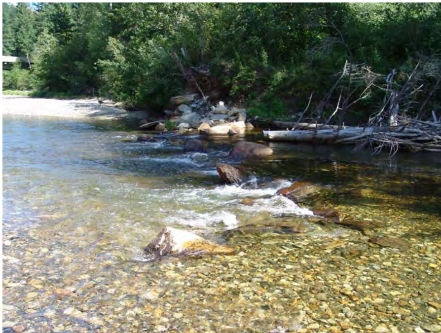
Photograph No. 3. View is to the east looking at an in-channel rock weir. Lower White Pine Reach; Subreach IZ-6, Nason Creek - Wenatchee Subbasin, Washington. Bureau of Reclamation Photograph by D. Bennett; August 8, 2007.
