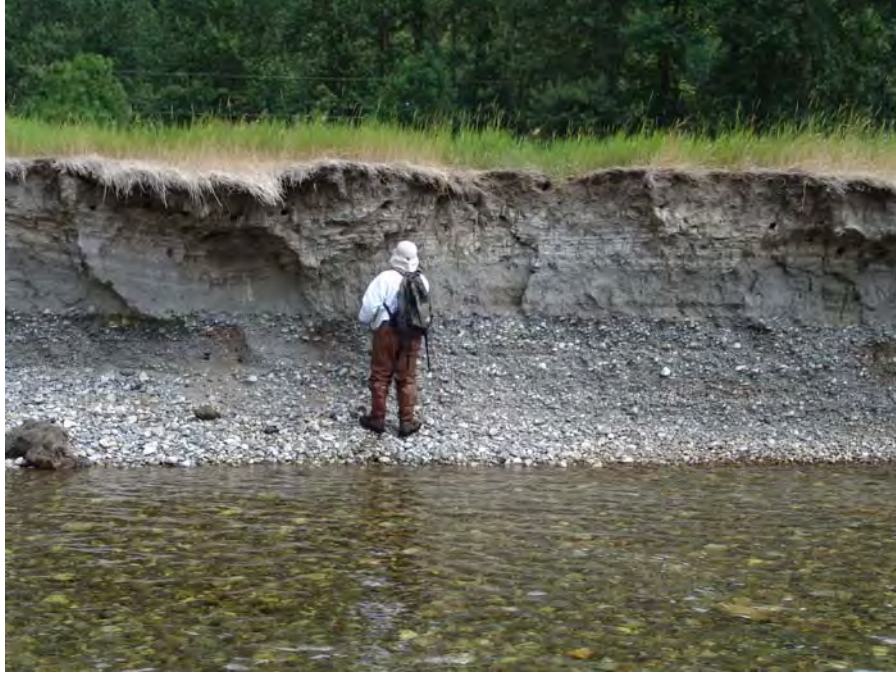
Photograph No. 2. View is to the north showing the stratified material in the left bank at a bank profile site. Lower White Pine Reach; Subreach IZ-2, Nason Creek - Wenatchee Subbasin, Washington. Bureau of Reclamation Photograph by D. Bennett; August 8, 2007.
