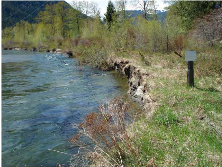
Photograph No. 3. View to the northwest looking upstream at brushy vegetation and the undercut/eroding along the left bank. Lower White Pine Reach; Subreach IZ-4, Nason Creek - Wenatchee Subbasin, Washington. Bureau of Reclamation Photograph by R. McAfee; May 3, 2007.
