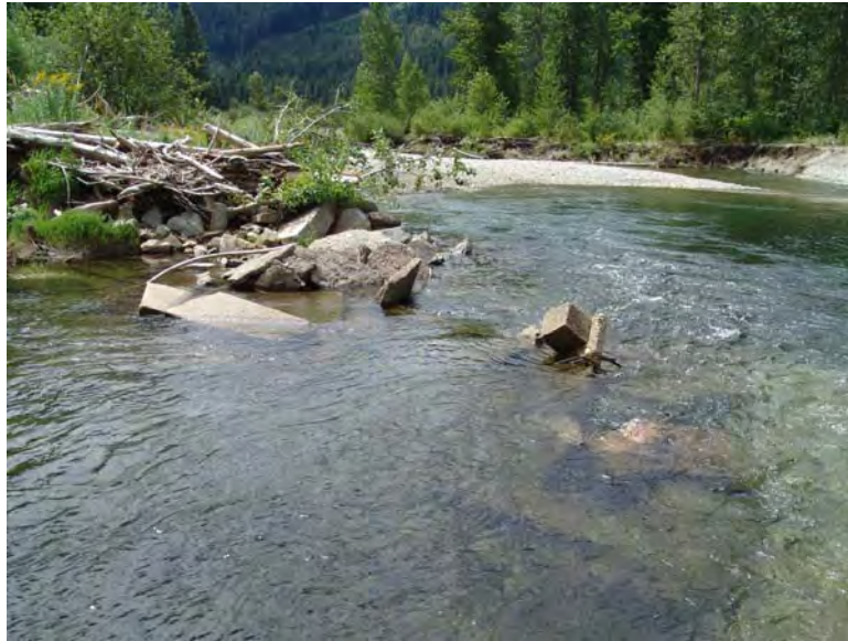
Figure 40 - In-channel structure comprised of concrete ecology blocks, miscellaneous concrete slabs and riprap, view to the south. Lower White Pine Reach; Subreach LWP IZ-4, Nason Creek - Wenatchee Subbasin, Washington. Bureau of Reclamation Photograph by D. Bennett; August 8, 2007.
