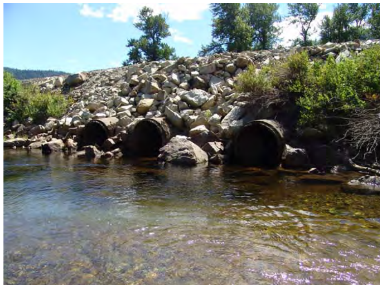
Figure 57 - Three concrete culverts that run through the railroad grade on the right bank, view is to the south. The culverts drain the area of LWP DIZ-2 and LWP DOZ-4. Lower White Pine Reach; Subreach LWP IZ-5, Nason Creek - Wenatchee Subbasin, Washington. Bureau of Reclamation Photograph by D. Bennett; August 8, 2007.
