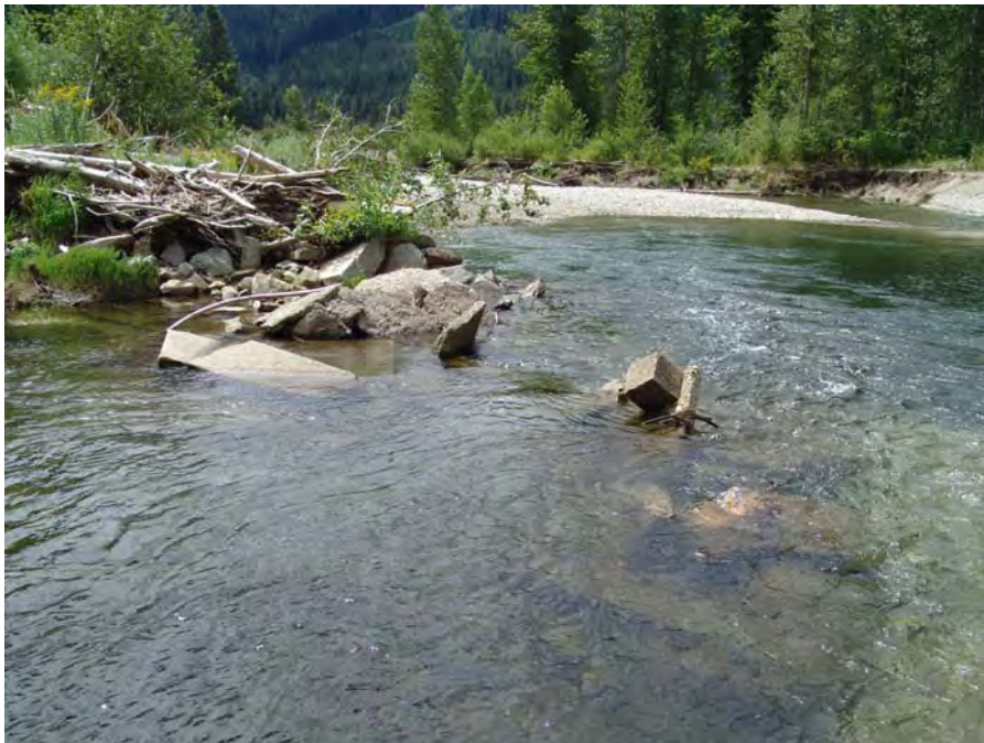
Photograph No. 7. View to the south looking at an in-channel structure comprised of concrete ecology blocks, miscellaneous concrete slabs and riprap. Lower White Pine Reach; Subreach IZ-4, Nason Creek - Wenatchee Subbasin, Washington. Bureau of Reclamation Photograph by D. Bennett; August 8, 2007.
