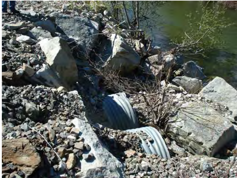
Figure 56 - Three elevated metal culverts that run through the railroad grade and drain the area of LWP DIZ-2 and LWP DOZ-4, view to the northwest. Lower White Pine Reach; Subreach LWP IZ-5, Nason Creek - Wenatchee Subbasin, Washington. Bureau of Reclamation Photograph by R. McAfee; May 4, 2007.
