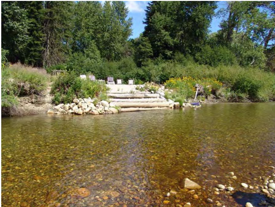
Photograph No. 17. View is to the north looking at small riprap and a constructed boat launch on left bank. Lower White Pine Reach; Subreach IZ-5, Nason Creek - Wenatchee Subbasin, Washington. Bureau of Reclamation Photograph by D. Bennett; August 8, 2007.
