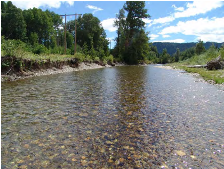
Photograph No. 5. View is to the southeast looking downstream at erosion along the left bank. Note the vegetation removal and a long run for the channel unit. Lower White Pine Reach; Subreach IZ-3, Nason Creek - Wenatchee Subbasin, Washington. Bureau of Reclamation Photograph by D. Bennett; August 8, 2007.
