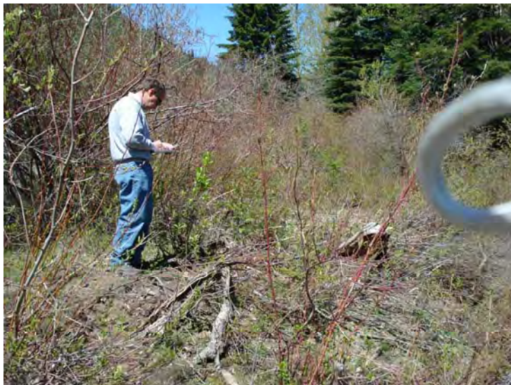
Figure 15 - Embankment on the left bank of the stream that cuts off a wetland area on the south side of the road in Subreach OZ-12, view to the northwest. Lower White Pine Reach, Nason Creek - Wenatchee Subbasin, Washington. Bureau of Reclamation Photograph by R. McAfee, May 3, 2007.
