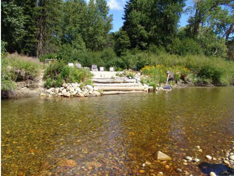
Figure 58 - Small riprap and a constructed boat launch on left bank, view is to the north. Lower White Pine Reach; Subreach LWP IZ-5, Nason Creek - Wenatchee Subbasin, Washington. Bureau of Reclamation Photograph by D. Bennett; August 8, 2007.
