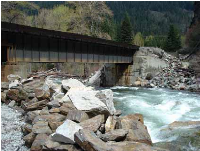
Figure 9. Downstream view to the north at riprap placed along USFS road and White Pine Railroad Bridge abutment near assessment area boundary (RM 14). (Reclamation photograph by R. McAfee, May 2, 2007).
