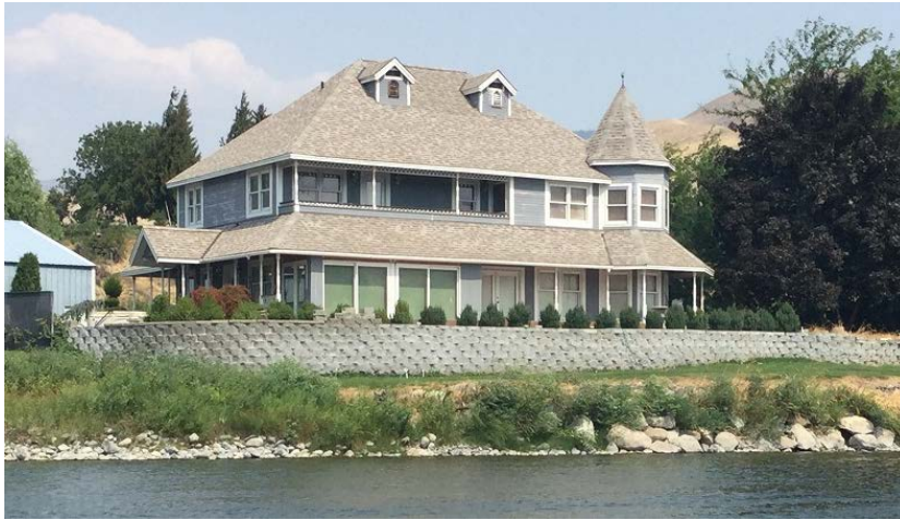
Figure 2-9. Example of Current Riverside Residential Development
