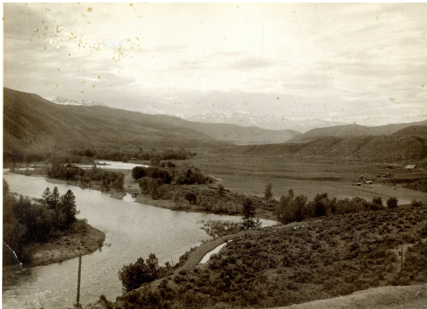
Figure 2-4. Historical (1904) Photograph from Chatham Hill Looking up the Wenatchee Valley into Sleepy Hollow Area (source: 1904 Photograph and Digital Image © Wenatchee Valley Museum and Cultural Center)
