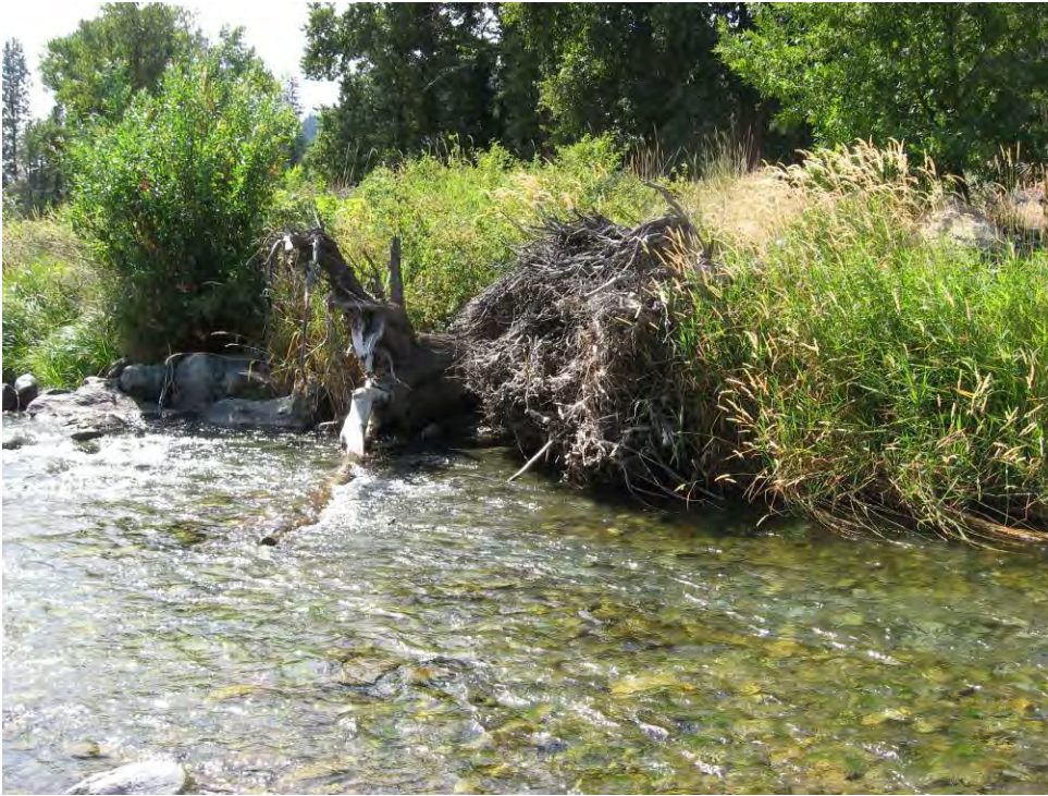
Figure 23. Logs with rootwads placed for streambank protection and fish habitat near river mile 4.2.
