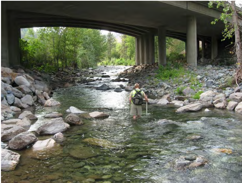
Figure 9. Hwy 97 Bridge at river mile 0.65.
