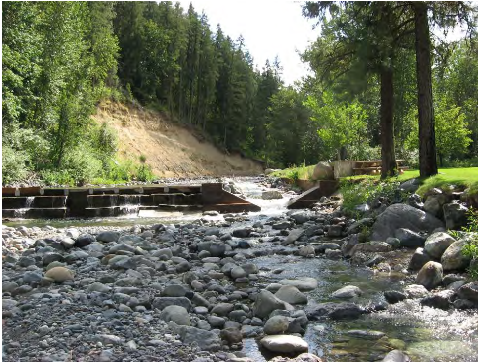
Figure 24. Irrigation diversion dam and fish passage channel at river mile 2.5.
