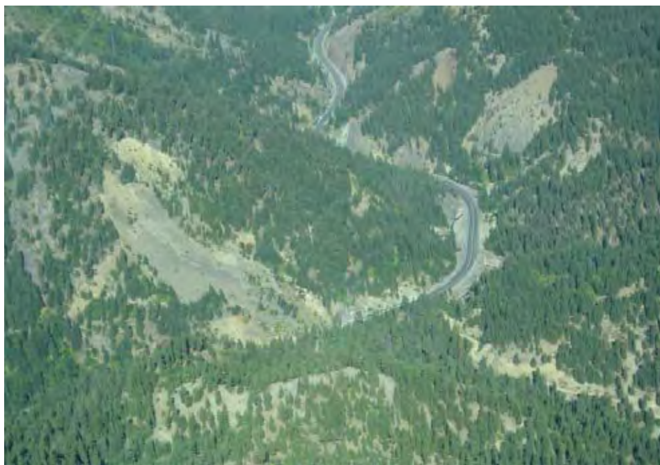
Figure 7. Low elevation aerial photo looking toward the northwest approximately 2.2 river miles upstream of the study area. The obvious slope instability on the left side of the photo is the Ruby Creek Slide.
