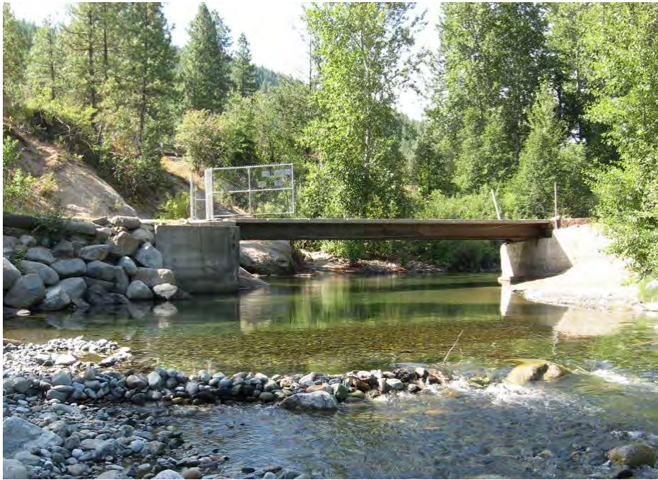
Figure 47. Private bridge crossing near river mile 6.5.
