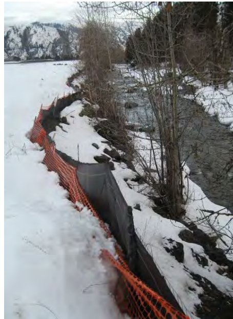
Figure 59. View looking downstream toward the northeast along the former Highway 97 road embankment. Rip-rap was left in place along this channel margin, and enhanced in some locations (January 2010).
