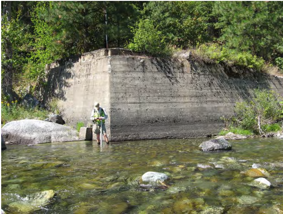
Figure 35. Concrete bridge abutment (no longer used) at river mile 5.3.
