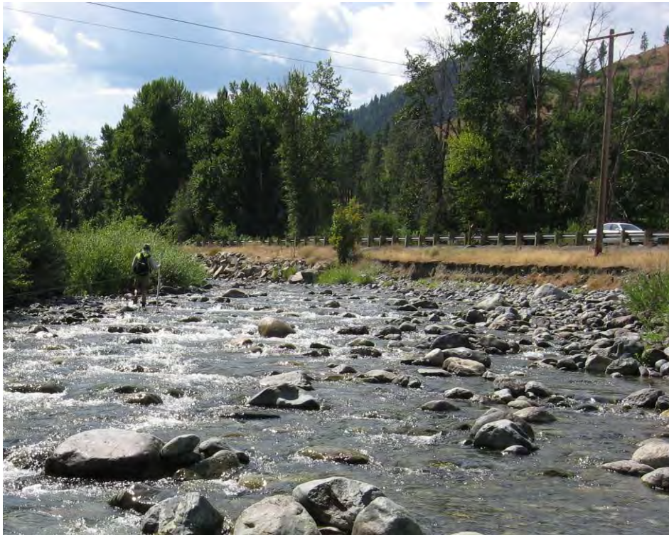
Figure 25. Impacted riparian corridor and rip-rap bank along Highway 97 near river mile 4.1 (river left bank).
