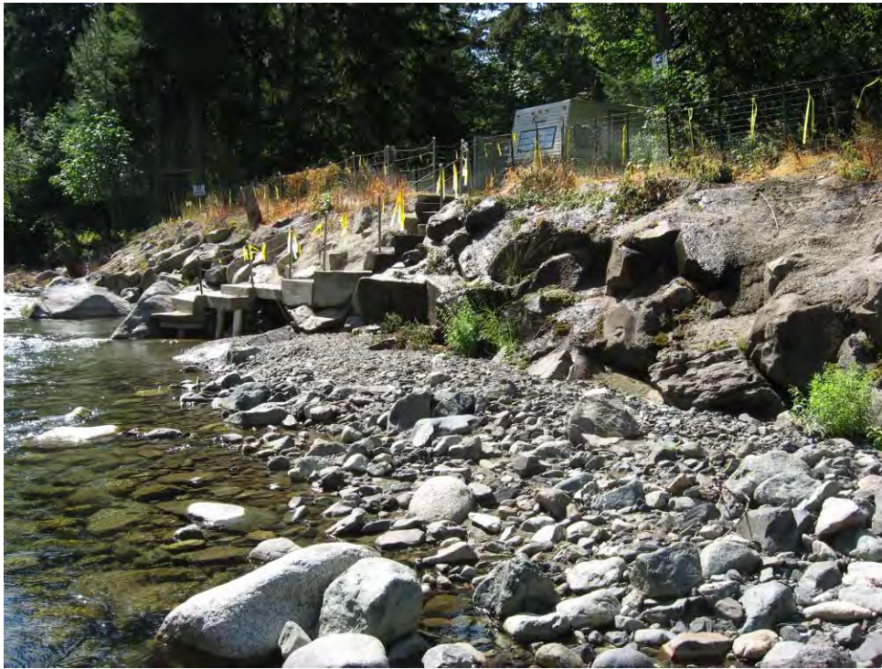
Figure 57. Bank armoring on river left bank near river mile 8.1.
