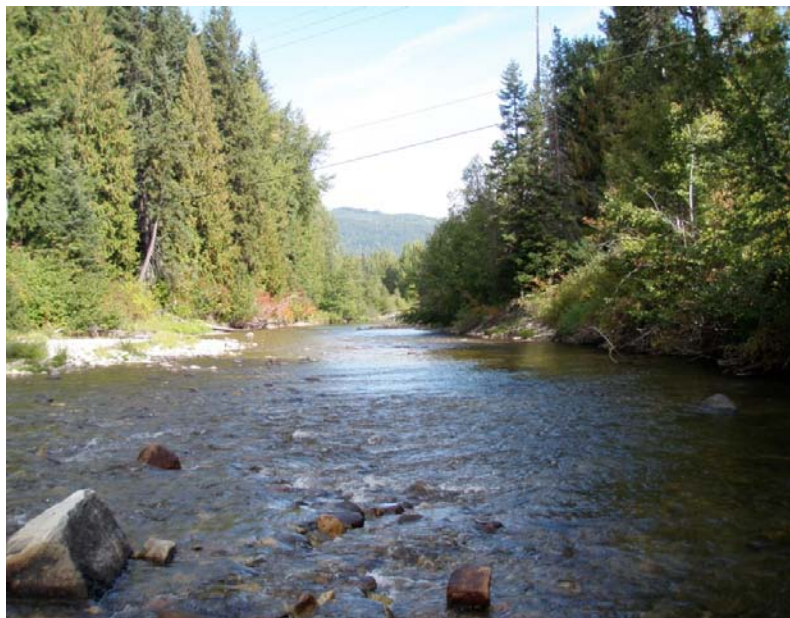
Figure 36. Channel Segment D: View looking downstream where the channel has been re-routed and confined by State Route 207 near RM 0.50. Lower Nason Creek, Wenatchee Subbasin, Washington – Bureau of Reclamation Photograph by E. Lyon, September 16, 2010.
