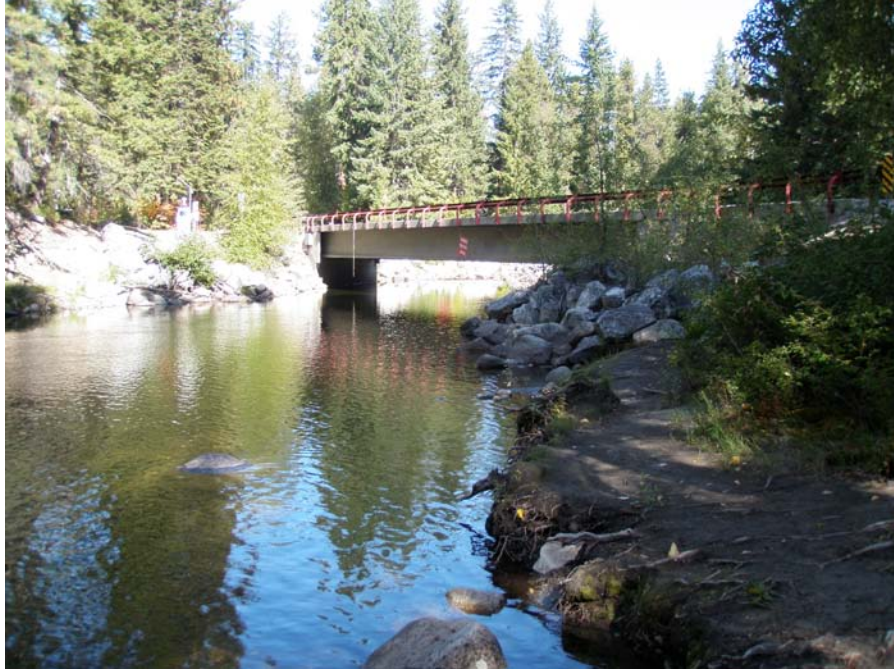
Photograph No. 3. View to the north looking at bridge crossing with riprap protecting abutments and artificially confining the channel. Lower Nason Creek, Wenatchee Subbasin, Washington – Bureau of Reclamation Photograph by E. Lyon, September 13, 2010.
