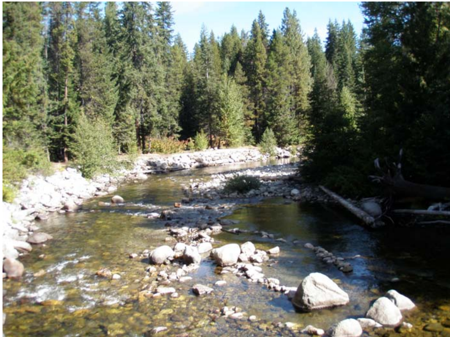
Photograph No. 4. View to the north looking from bridge crossing downstream at riprap protecting campground along river left. Lower Nason Creek, Wenatchee Subbasin, Washington – Bureau of Reclamation Photograph by E. Lyon, September 13, 2010.
